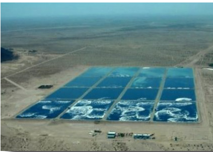
Las Arenitas Wastewater Treatment Plant in Mexicali
