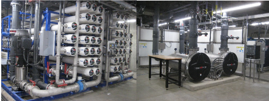
On the left: Reverse Osmosis (RO) Trains; on the right: Ultra-violet (UV) treatment trains
