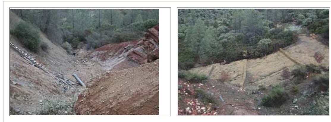
Alpine Millsite before and after cleanup and restoration
