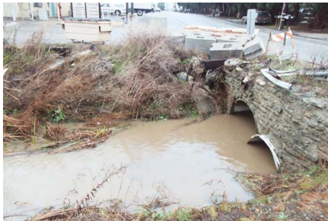
Figure 6.9 Watsonville Slough at Lee Rd. (Photo: F. Watson Dec 02).
