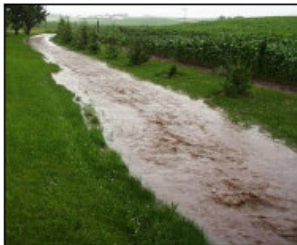
No problem for a 3 foot wide swale !
