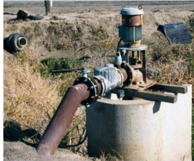
Figure 7. Control (butterfly) valve, air-vacuum relief valve, and check valve located downstream of tailwater return pump. Photo: Lawrence J. Schwankl.
