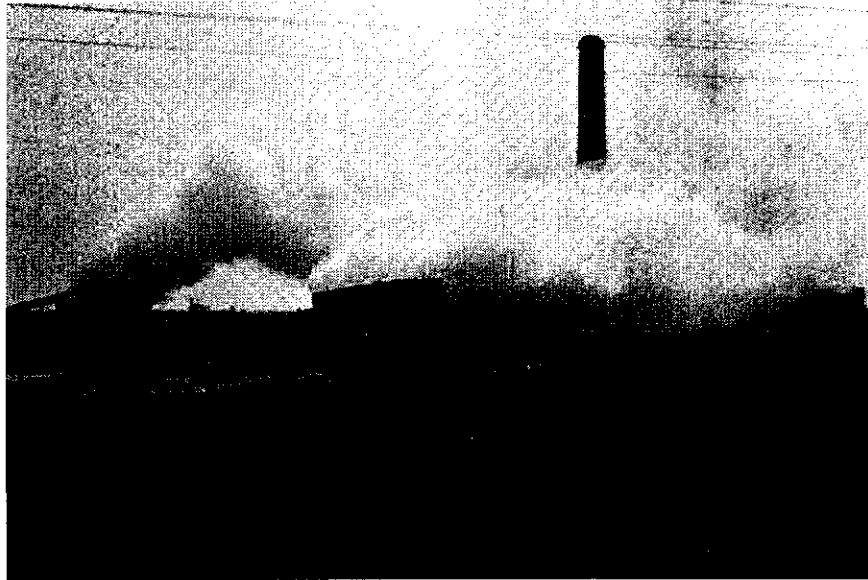
Figure 7- Plume of a Modest Wet Mechanical Draft Cooling Tower
