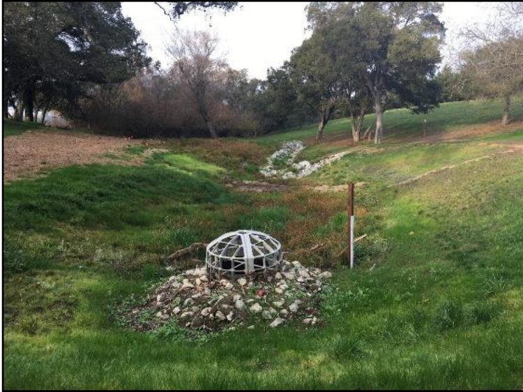
Figure 4-6. Constructed sediment basin captures agriculturally derived stormwater and return flows from multiple farms near Pinto Lake (photo credit: City of Watsonville and the RCDSCC).
