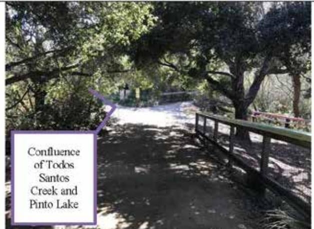
After Photo: Gully has been filled and road has been sloped to address future surface flows. (Direction: Looking West)
