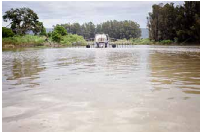
Photo 15 HAB Aquatic Solutions, LLC. barge dosing Pinto Lake with alum, April 2017 [Credit: Catherine Bosley, HAB Aquatic Solutions, LLC.]
