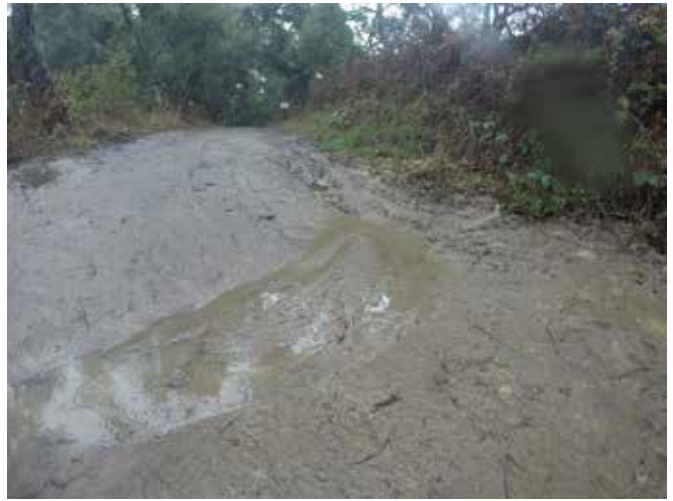
Photo 24 The implemented rolling dips in action, moving water off the access road to inhibit downcutting, October 28, 2016
