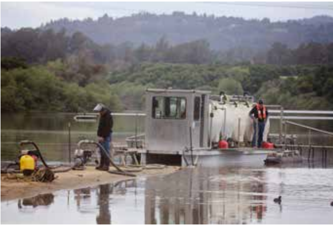
Photo 14 HAB Aquatic Solutions, LLC. staff prepare the barge for alum treatment at Pinto Lake, April 2017 [Credit: Catherine Bosley, HAB Aquatic Solutions, LLC.]
