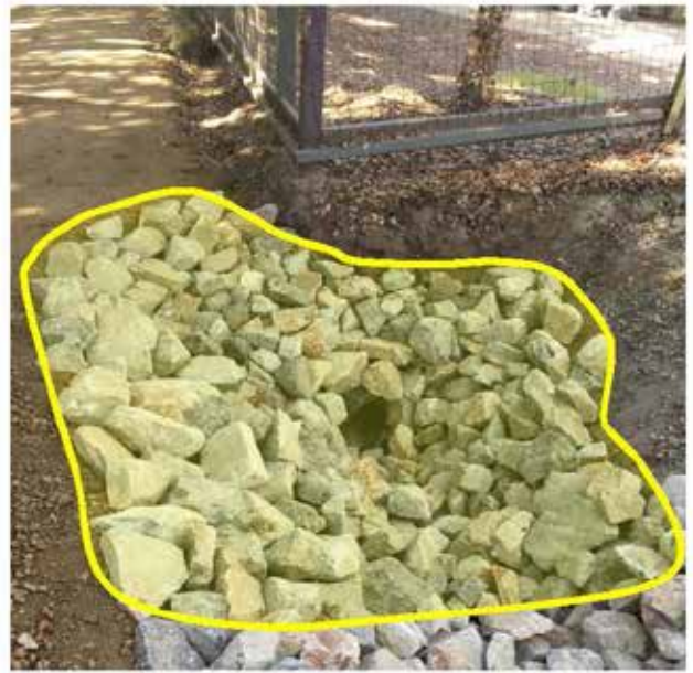
After Photo: Culvert inlet location. (Direction: Looking West)
