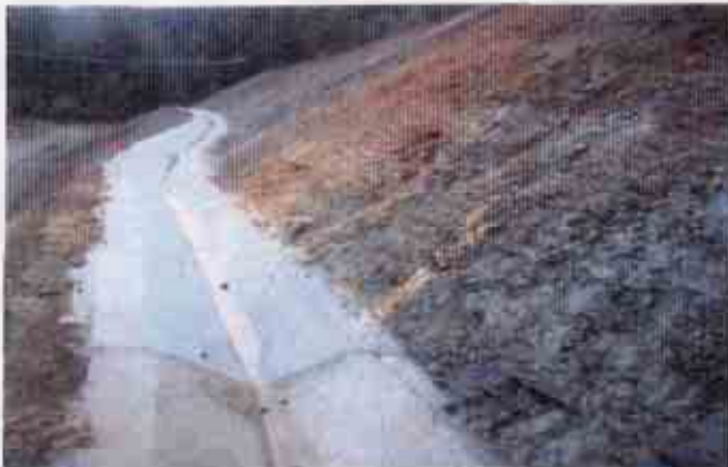
Figure 1: One of the many areas where soil is slumping on the steep slopes on the northern side of the project
