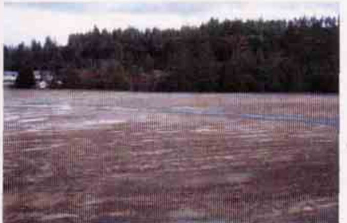
Figure 18: Lack of an effective combination of erosion and sediment control BMPs
