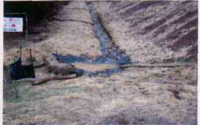
Figure 8: Turbid storm water flowing down to the western discharge location
