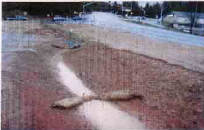
Figure 33: Turbid storm water discharging from the project
