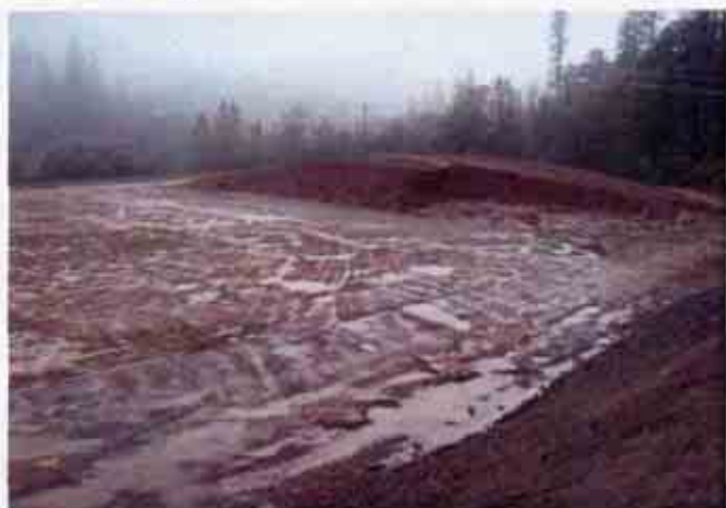
Figure 3: Overview of another portion of the project
