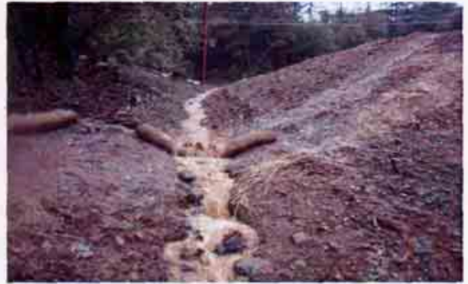
Figure 14: Discharge from the site cutting into the bank on the western side of the project.
