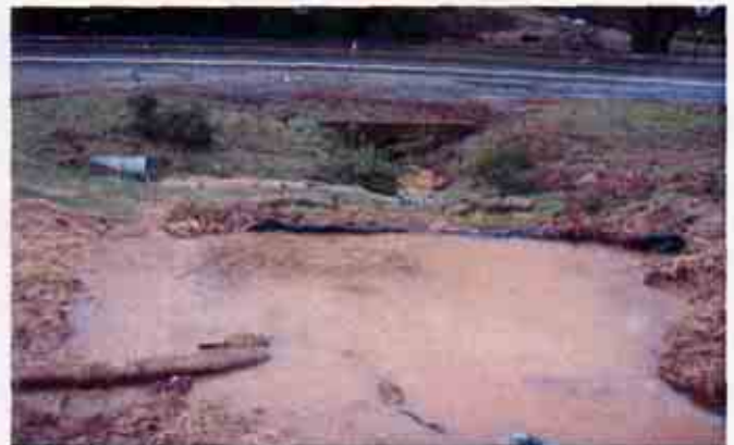
Figure 16: Very turbid storm water from the site discharging into the western culvert.
