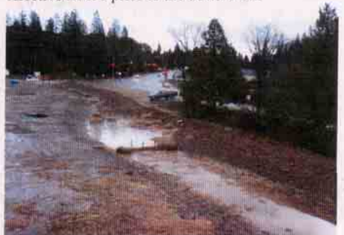
Figure 22: Turbid storm water ponded onsite
