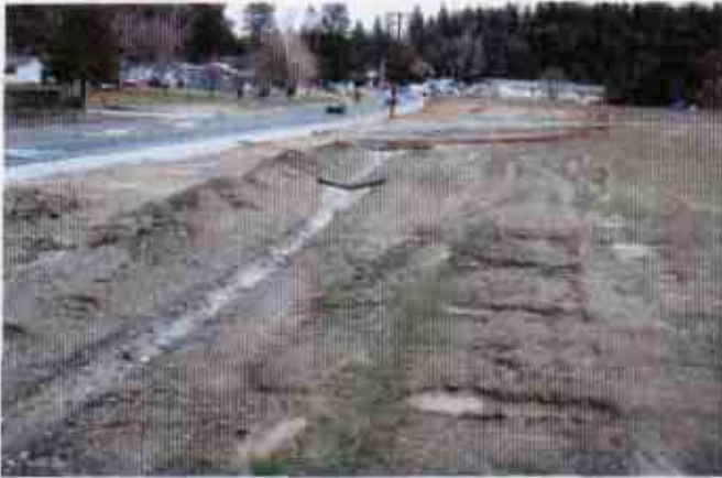
Figure 7: Poor erosion control BMPs
