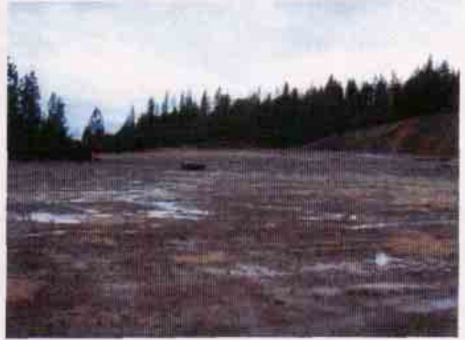
Figure 32: Lack of an effective combination of erosion and sediment control BMPs
