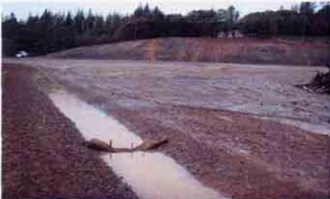
Figure 3: Another view of a portion of the project. Note the lack of BMPs.
