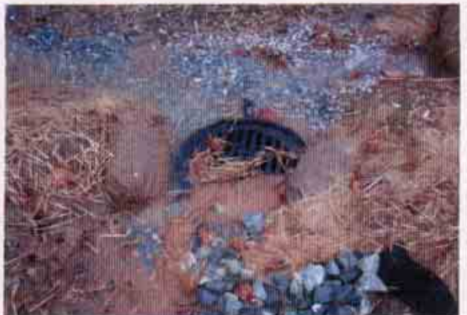
Figure 30: Another view of the drain inlet along Ridge Road
