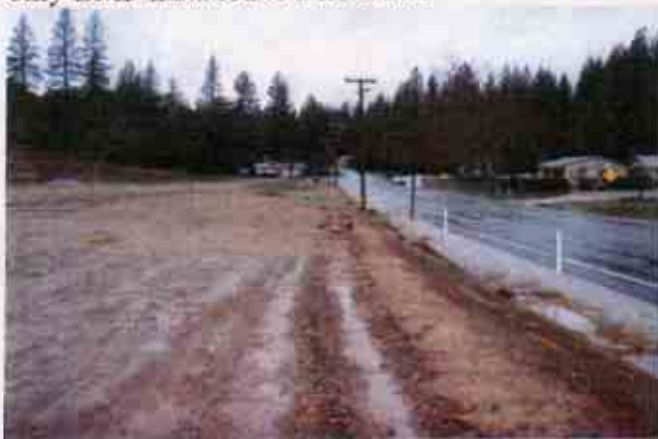
Figure 27: Light application of straw mulch along Ridge Road
