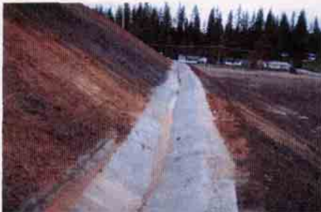
Figure 17: Turbid storm water in the concrete channel that runs along the slope on the northern side of the project
