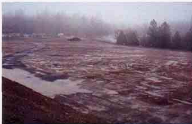
Figure 2: Overview of one portion of the project
