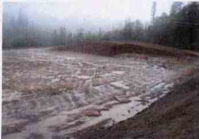
Figure 3: Overview of another portion of the project
