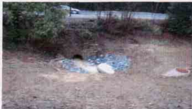
Figure 15: Storm water discharge from the site entering the culvert which flows under the highway and directly into the creek
