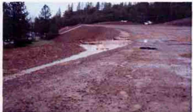
Figure 6: Turbid storm water discharging into the culvert.
