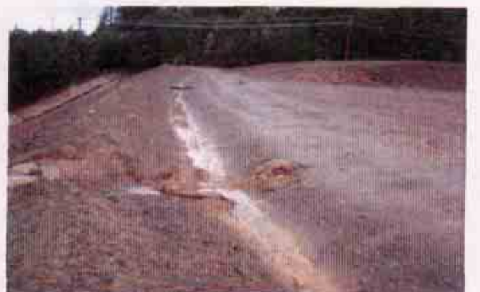
Figure 18: Another view of the fiber rolls installed prior to discharge into the down drain
