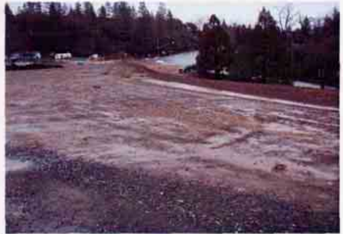
Figure 8: Another portion of the project without effective storm water management BMPs.
