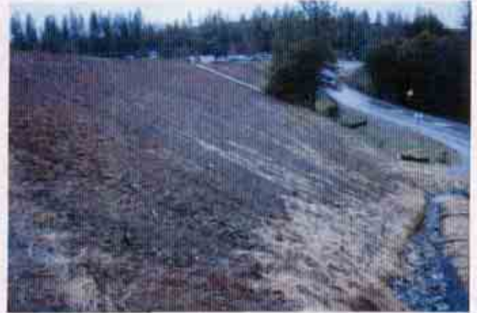
Figure 8: Same area Note: the general lack of BMPs on the slope
