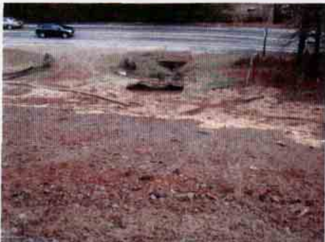
Figure 5: Rilling on the slope
