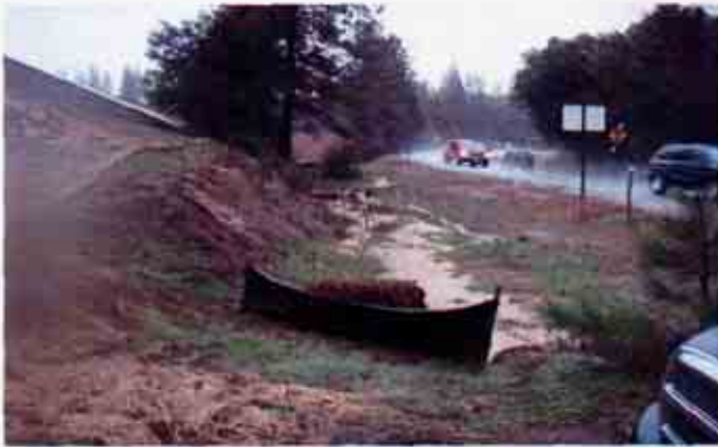
Figure 13: Discharge from the site flowing along the Highway 88 right of way.
