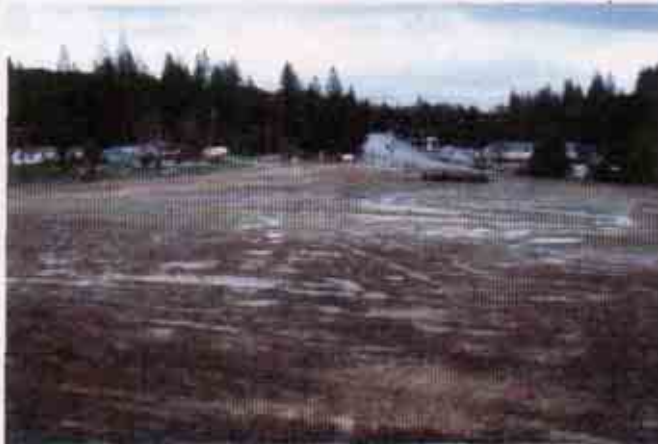
Figure 19: Lack of an effective combination of erosion and sediment control BMPs
