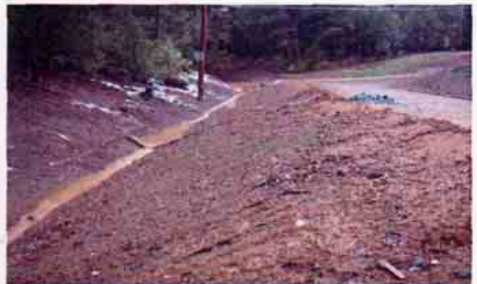
Figure 12: Partially stabilized slope on the western side of the project.
