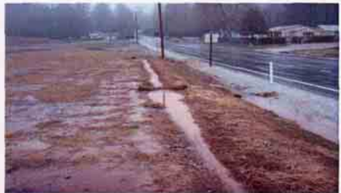
Figure 16: Storm water flowing on the site along Ridge Road
