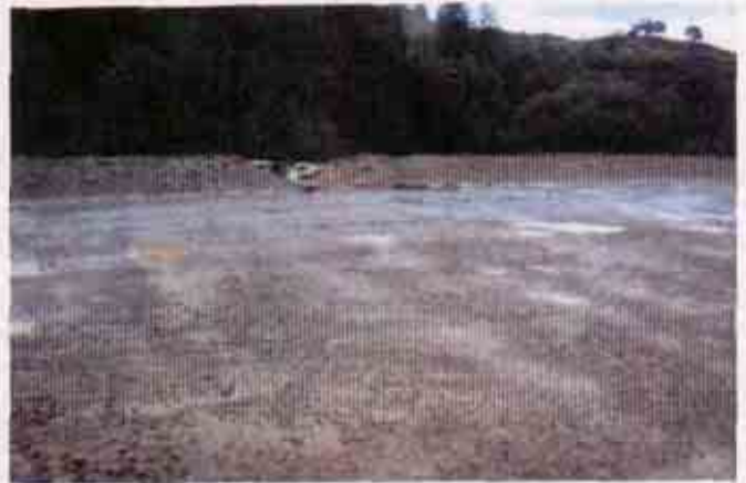
Figure 26: Lack of an effective combination of erosion and sediment control BMPs around one of the discharge locations
