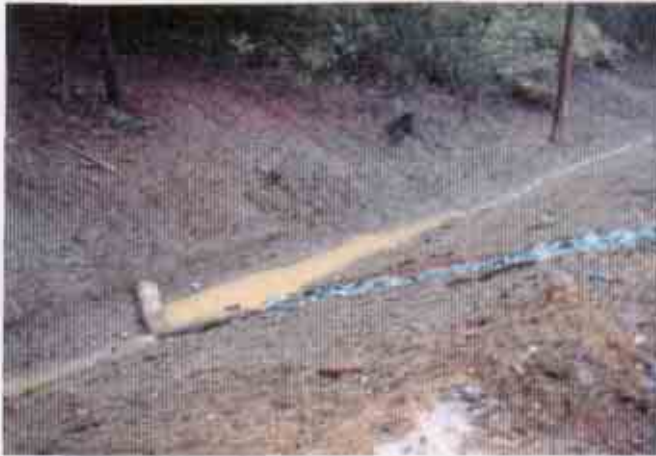
Figure 7: Lack of an effective combination of erosion and sediment control BMPs
