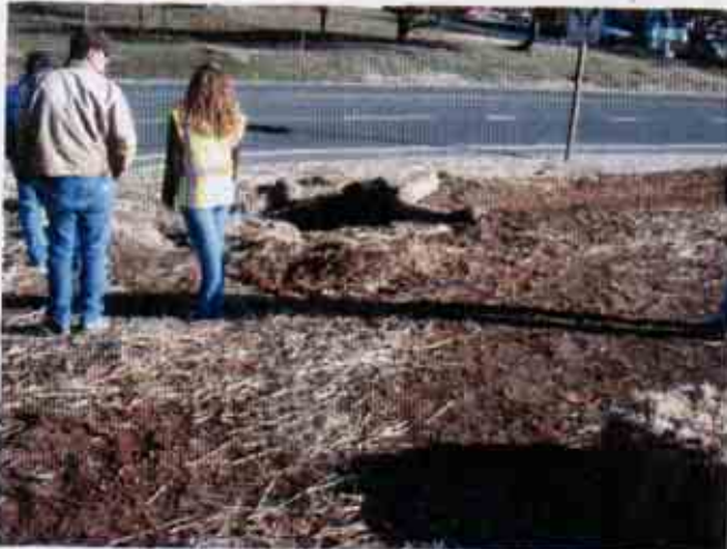
Figure 9: Another view of the poorly protected drain inlet
