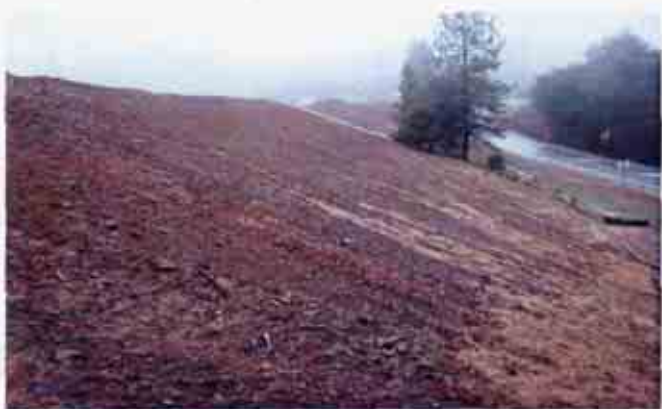
Figure 9: Poorly protected slopes
