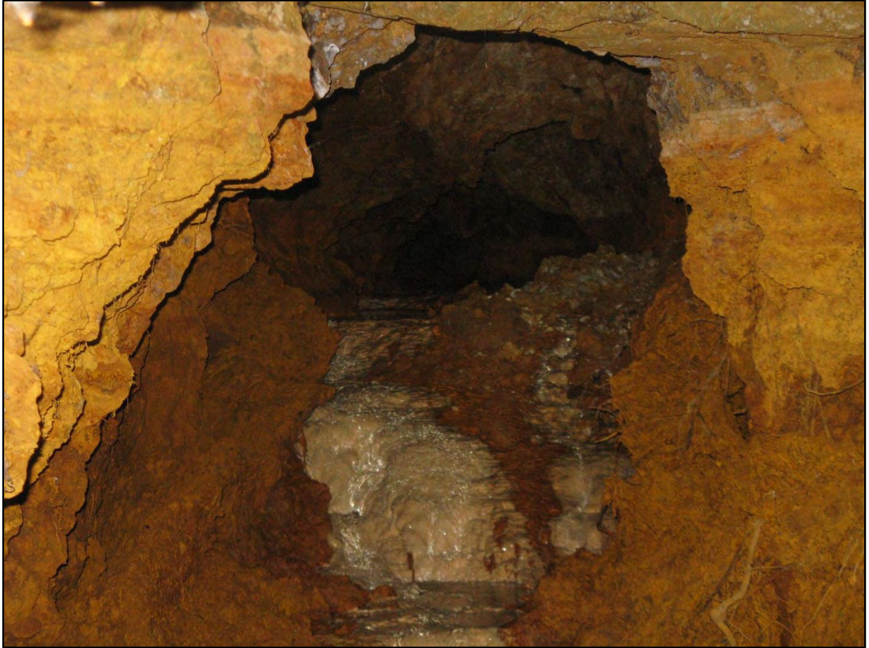
Figure 17. Interior of Twin Peaks Mine Adit 3 showing running water and a relatively narrow and low channel.
