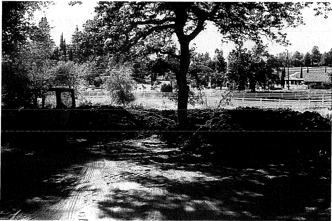
Figure 6. View of stockpiled excavated soil on project site.
