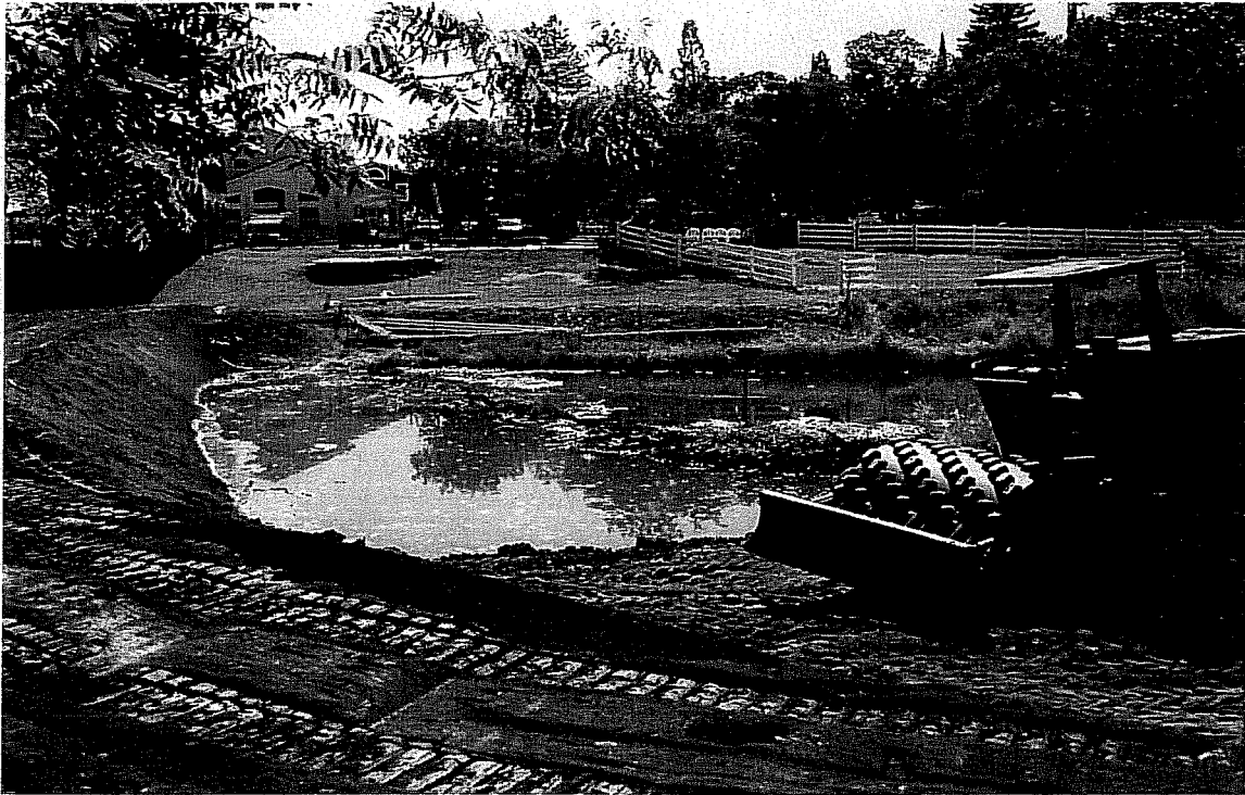
Figure 3. View of illegal impoundment on north side of drainage. Poned section.
