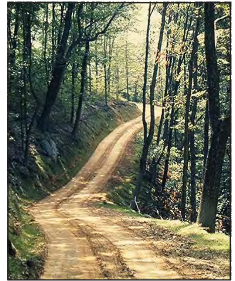
Photo 4.2 Locate roads to conform to the natural terrain and roll the road grades to disperse surface water frequently.
