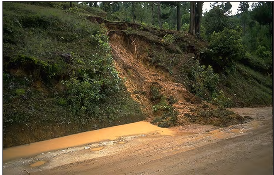
Photo 4.11 Remove slide material that blocks the drainage ditches and narrows the road.
