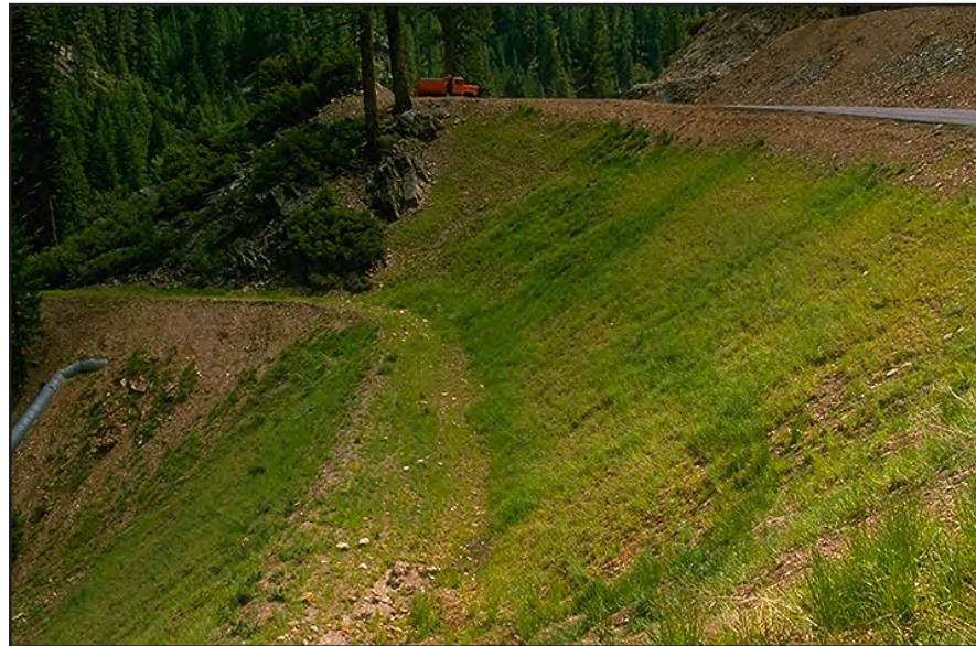
Photo 11.5 Construct fill slopes with a 1 1/2:1 or flatter slope (to promote vegetation growth) and stabilize the fill slope surface. Use benches (terraces) on large fill slopes to intercept any flow of surface water.
