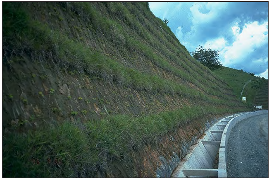
Photo 13.10 Use of grasses, planted on contour, to provide surface slope stabilization and erosion control on a steep road cut.
