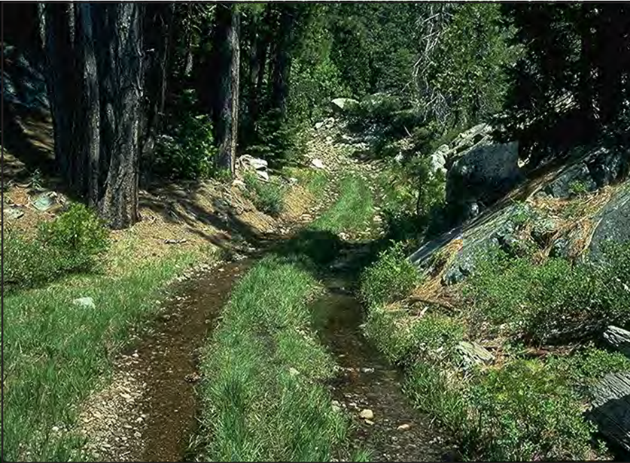
Photo 3.2 A poor road location where the road has become a “creek” and is hydrologically “connected” to streams around it.
