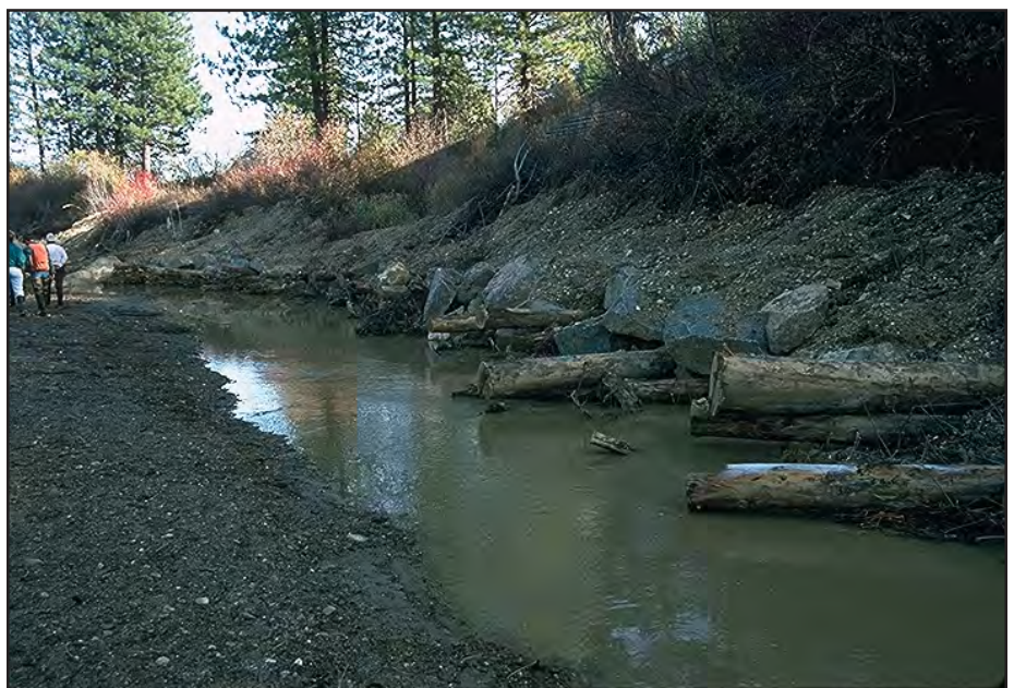
Photo 6.3 A root wad, log, and rock armored stream bank built for protection against scour. Logs and vegetation can offer an attractive alternative to riprap in relatively low stream velocity areas.
