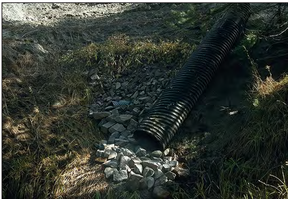
Photo 8.1 Protect the outlet of culverts against erosion. Graded riprap is common for this purpose.
