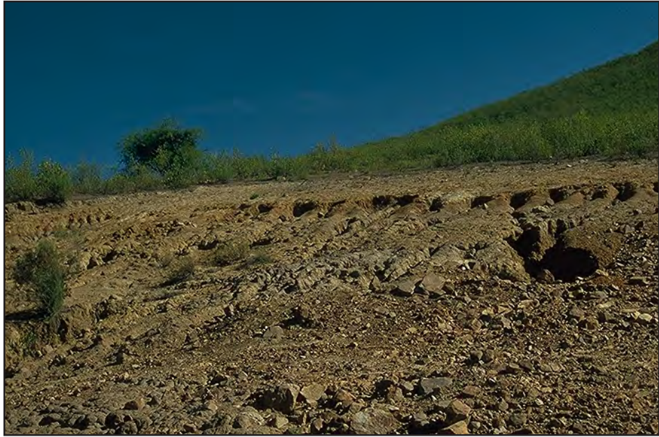
Photo 12.11 This roadside borrow area lacks drainage and erosion control. Roadside quarry development can be inexpensive and useful, but the areas should be hidden if possible, and the areas should be reclaimed once the project is completed.
