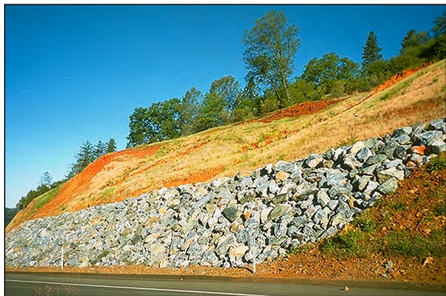
Photo 11.7 A drained rock buttress can be used to stabilize a cut slope failure area.
