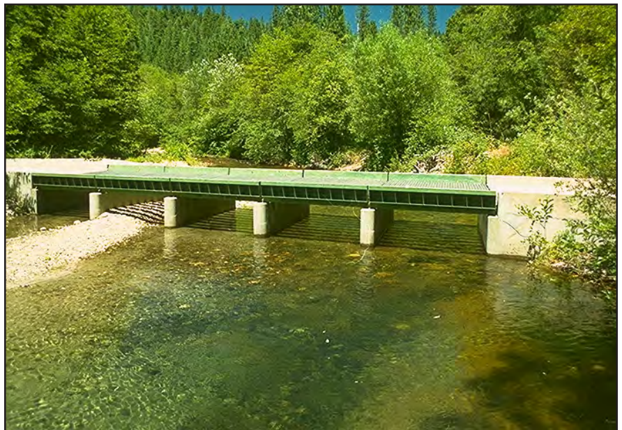
Photo 9.5 Some fords can be designed as “low-water bridge” structures. They must be designed to be occasionally overtopped and have an erosion resistance deck and approaches. This structure is ideal for fish passage.
