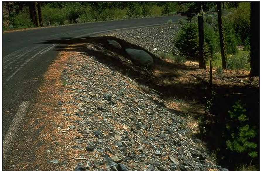
Photo 13.7 Rock armoring, placed on a very erosive soil fill slope adjacent to a creek, used for durable, permanent erosion control.
