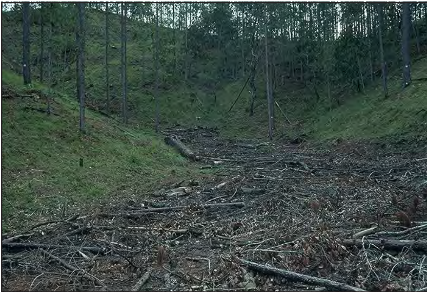
Photo 13.4 A disturbed work area covered with woody material such as brush from clearing or logging slash for erosion control . Ensure that the material is well mashed onto the ground.
