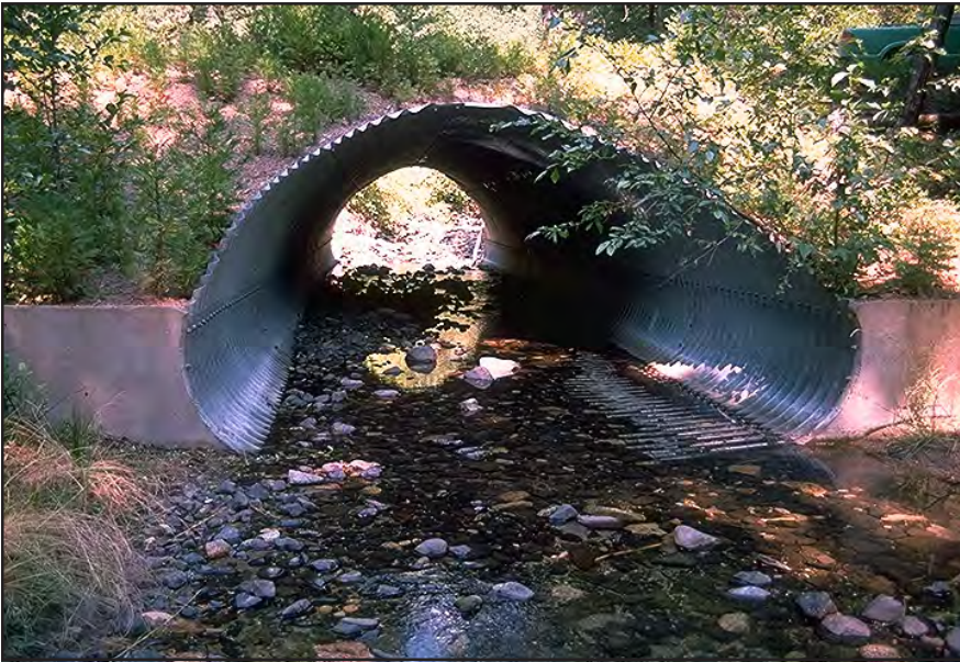
Photo 8.7 Use structures with natural stream bottoms, such as arch pipes, bottomless arches, or concrete box culverts, to promote fish passage and minimize impacts to the stream.
