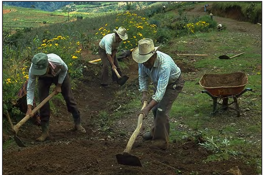
Photo 4.9 Perform road maintenance, either with equipment or by hand, to keep the roadway shaped and drainage structures functioning. Keep ditches clean but do not remove the layer of vegetative (grass) stabilization.
