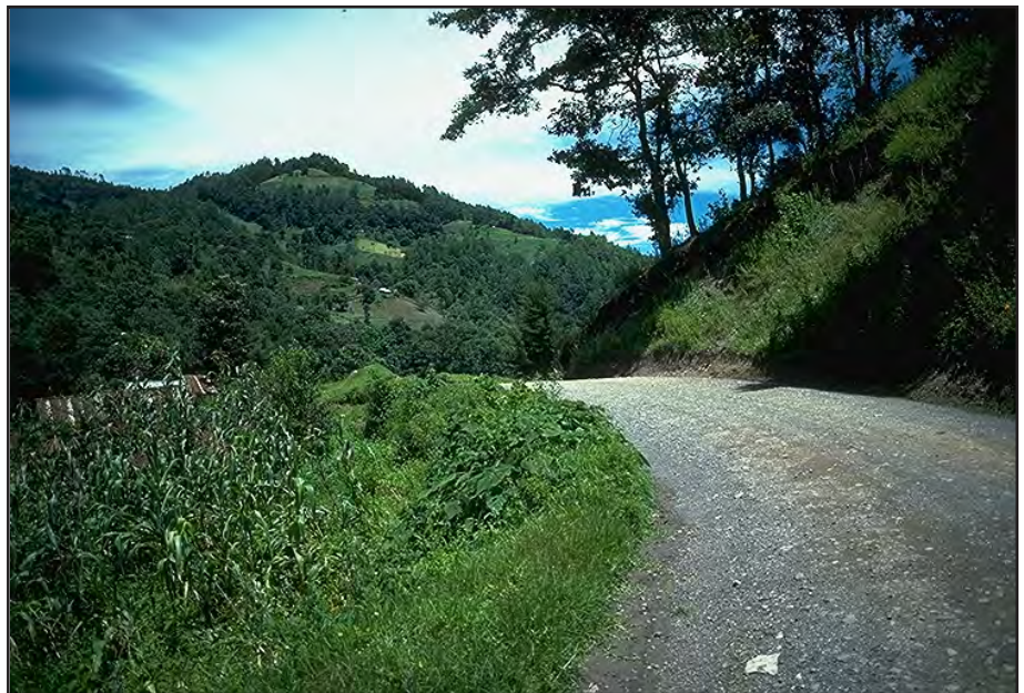
Photo 2.5 A well designed, “minimum impact” road that has an appropriate standard for its use, good drainage, and stable slopes.
