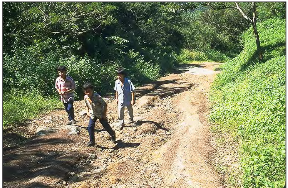
Photo 2.4 Adverse environmental impact from road surface erosion caused by steep road grades and insufficient cross-drains. This road is also difficult to maintain.
