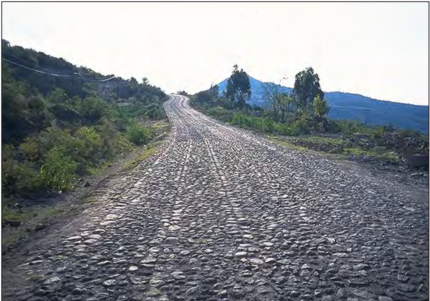
Photo 1.4 A well designed, “minimum impact” road that has an appropriate standard for its use, and a stabilized cobblestone driving surface.
