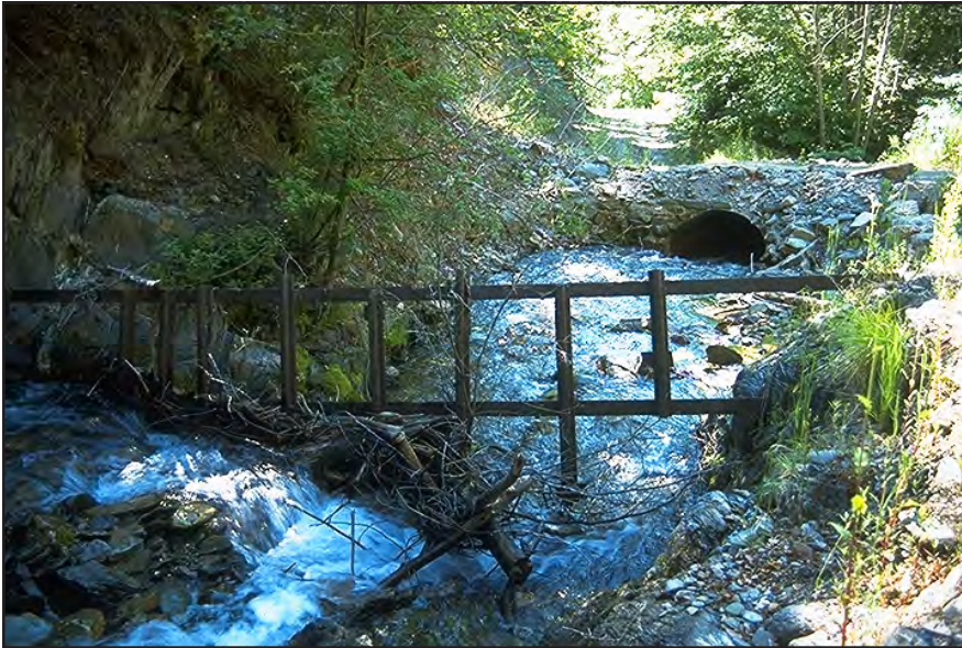
Photo 8.5 Use trash racks on culverts where a lot of debris is found in the channel. Remember that trash racks require cleaning and maintenance.
