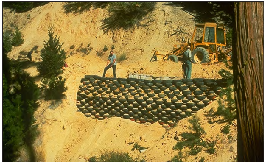
Photo 11.10 A road fill failure in steep terrain which now needs either a retaining structure or a large road cut around the failure.
