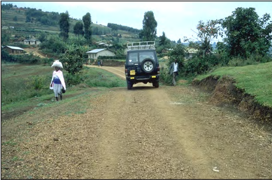
Photo 2.1 A well built road that helps serve the local population in a rural area, with minimum environmental damage.
