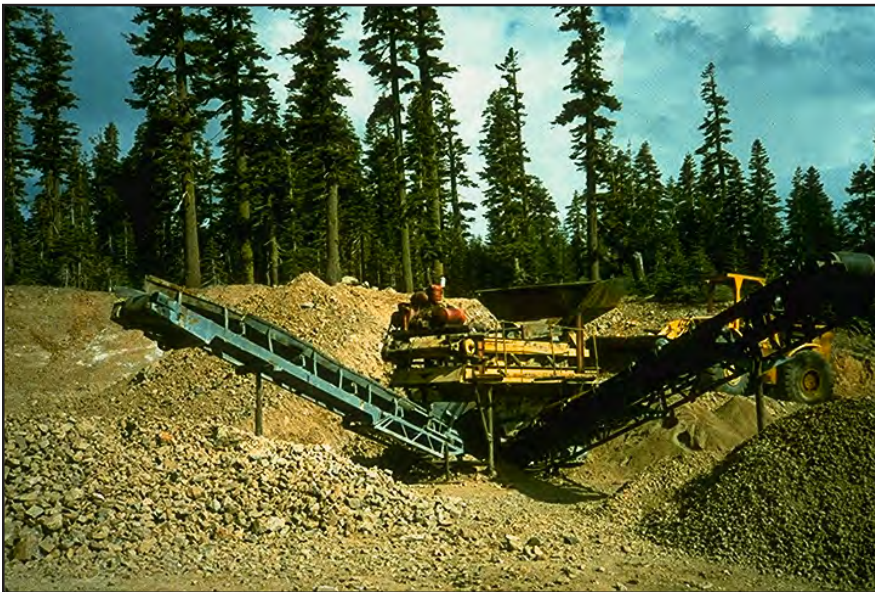
Photo 12.10 Quarries and borrow sites (materials sources) can provide an excellent, relatively inexpensive source of project materials. A site may require simple excavation, screening, or crushing to produce the desired materials. Control use of the area with a Pit Development Plan.
