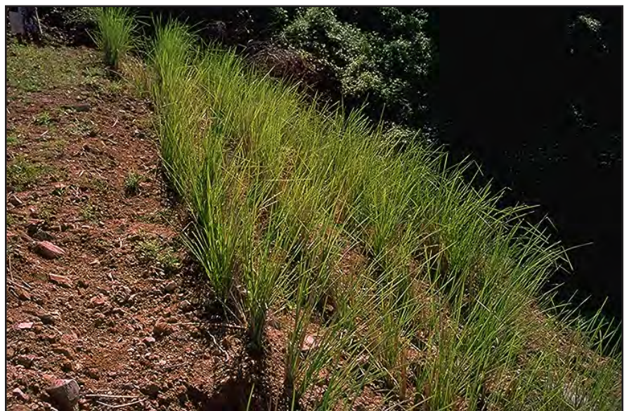
Photo 13.9 Use of Vetiver grass for slope stabilization and erosion control. Choose vegetation that is adapted to the site, has strong roots, and provides good ground cover. Ideally, use native species.
