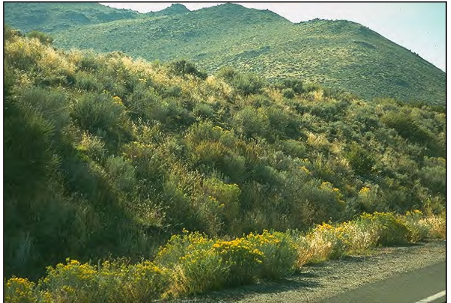
Photo 11.3 A well-stabilized cut slope, with about a 1:1 slope, that is well covered with vegetation.
