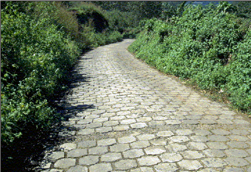
Photo 12.7 Concrete blocks (Adoquin) or cobblestone offer an intermediate alternative to aggregate and pavement road surfacing. These materials are labor intensive to construct and maintain, but are very cost-effective in many areas.
