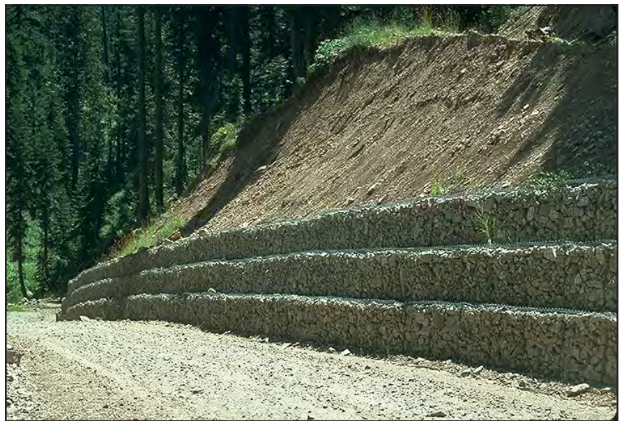
Photo 11.9 Gabions are a commonly used type of low gravity retaining structure because they use locally available rock and are relatively inexpensive.
