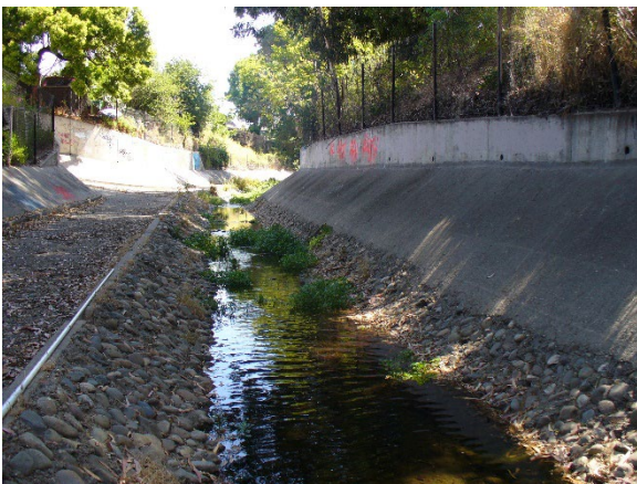
Figure 32. Examples of reaches with two hardened banks. Left: San Leandro Creek (Alameda County). Right: Morrison Creek (Sacramento County).
