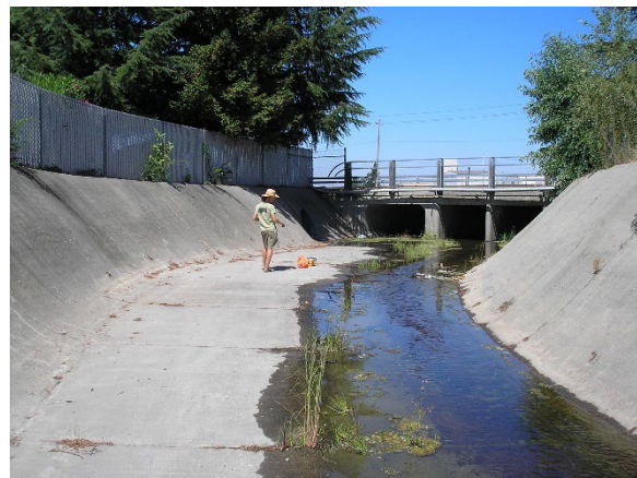
Figure 32. Examples of reaches with two hardened banks. Left: San Leandro Creek (Alameda County). Right: Morrison Creek (Sacramento County).
