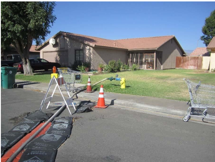
Photo 1. 2013 temporary intertie with IWA.
