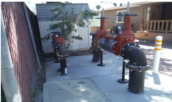
Photo 1 Finished installation of backflow prevention pipe.
