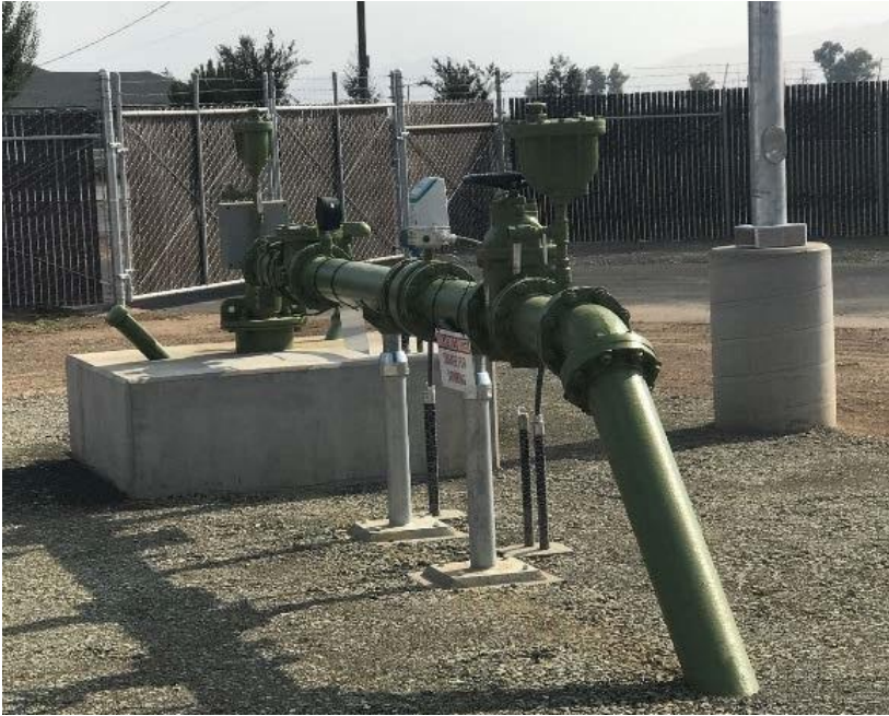
Photo 2 New well head.
