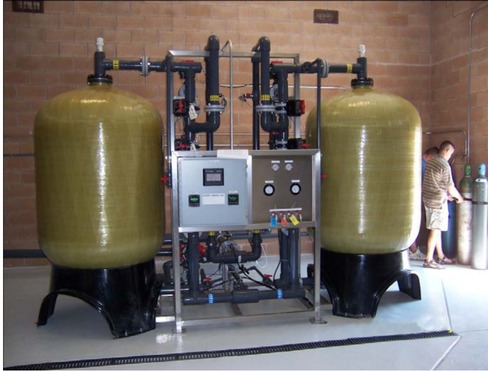
Figure 2-1E. 160-gpm E33 Media Arsenic Adsorption System by AdEdge (Two FRP Vessels in Parallel)
