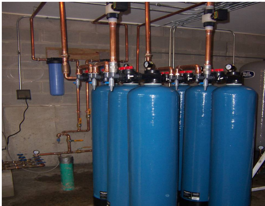
Figure 2-1B. 14-gpm As/I Complex 2000 Media System by ATS (Two Trains of Three Polyglass Vessels in Series)
