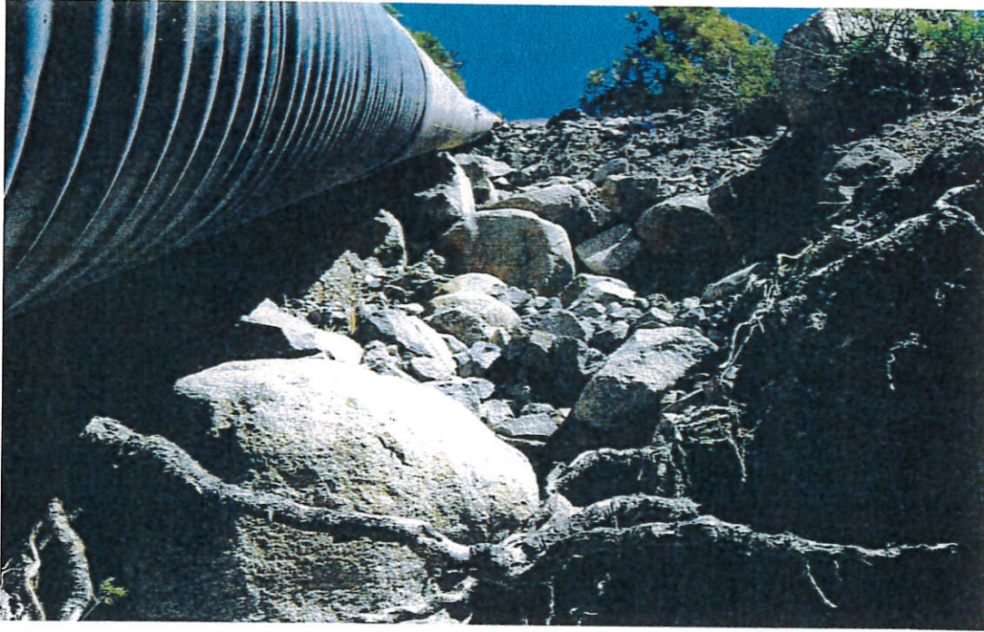
Photo 1. Looking upslope along at the Caltrans culvert on the east end of the hillside above West Reed Avenue. Photo taken June 6, 2006.
