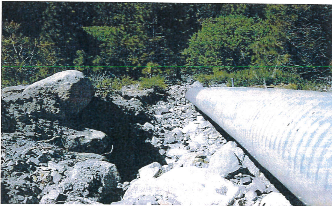
Photo 2. Looking downslope along the culvert where eroded material is being transported down the hillside above West Reed Avenue. Photo taken June 6, 2006.
