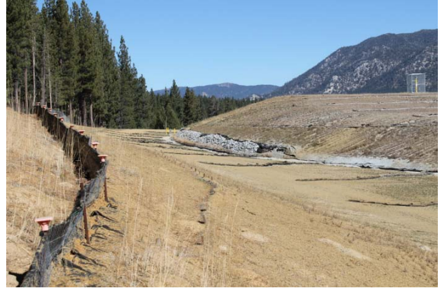
Rock-armored base of slope above channel, tackifier, straw waddles and revegetation
