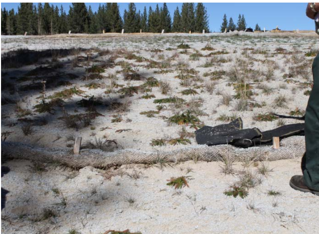
Area with bare soil & flattened straw waddle
