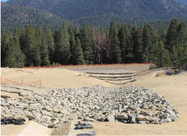
Condition in October 2013 after repairs
