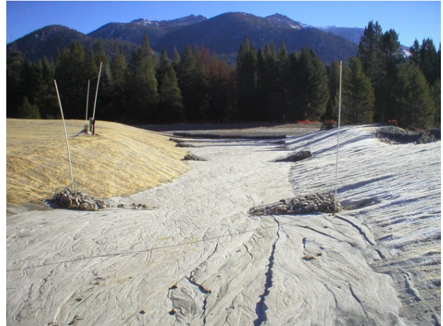
Condition after December 2012 storm event
