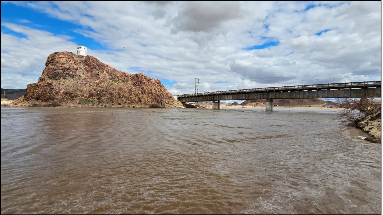
Figure 3.4 - Barstow First Street from west side of the First Street Bridge on 03/23/2023. USGS Barstow stream gage measured discharge 308 cubic feet per second
