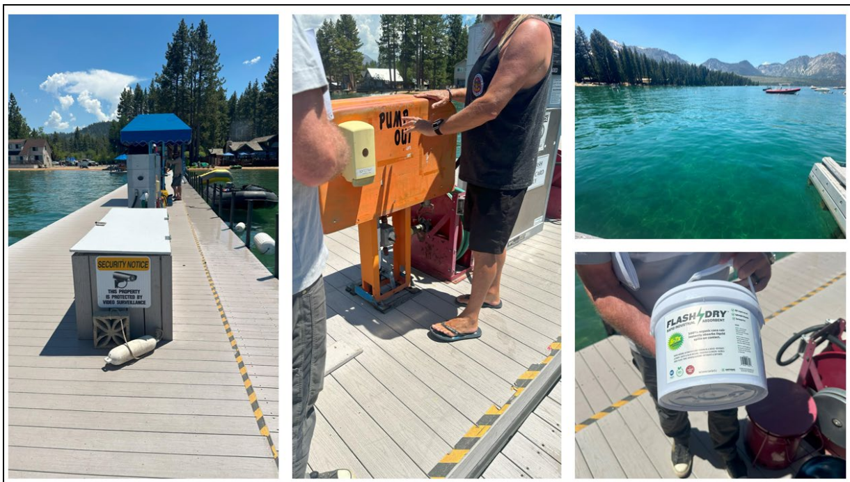
Photo 5.1: Camp Richardson Marina inspection, from left, fueling and emergency spill kit location, sewage pump out (not in use), water adjacent to marina, one of several spill kits for emergency use. Photos taken June 13, 2024.
