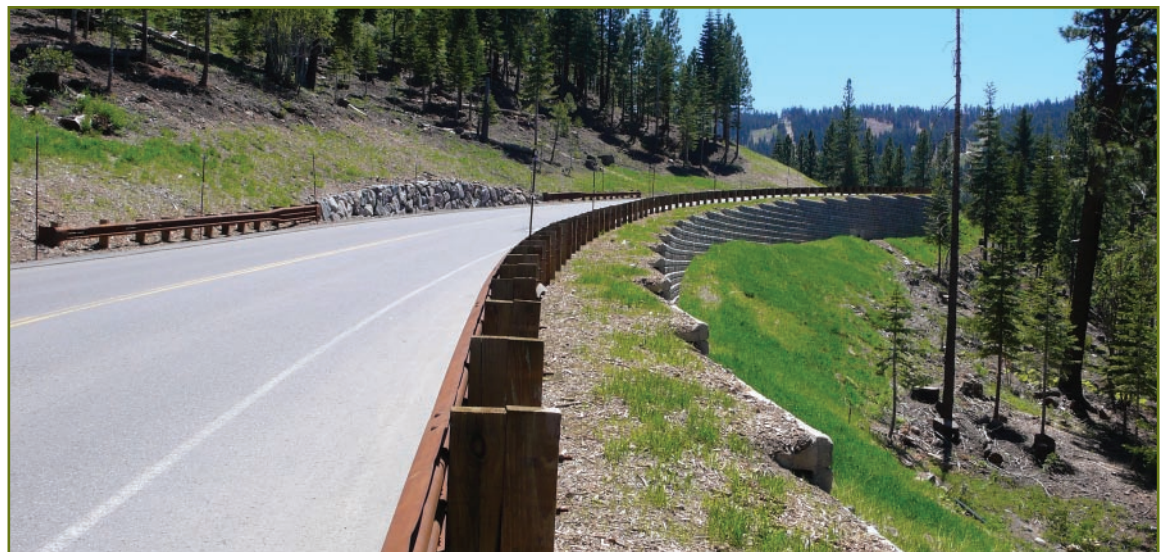
Highlands View Road at Northstar-at-Tahoe, one year following treatment. Topsoil was salvaged and re-applied along 4 miles of cut-and-fill slopes.
