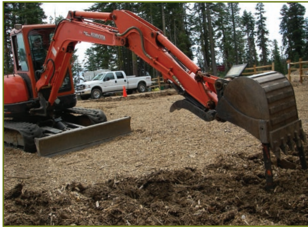
Infiltration tines mounted on excavator bucket being used to loosen soil and incorporate wood chips.
