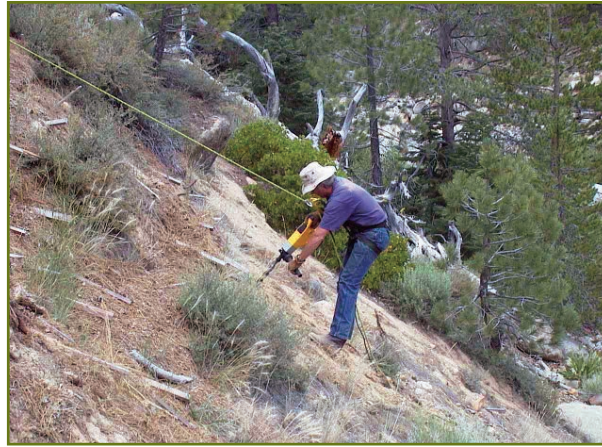
2- Drilling holes in slope with hammer drill.
