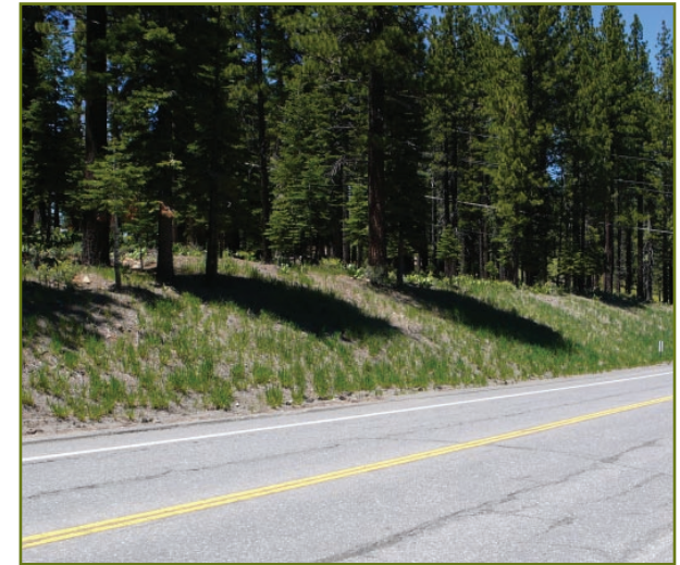
Repaired slope exhibiting long-term stability – Summer 2008.
