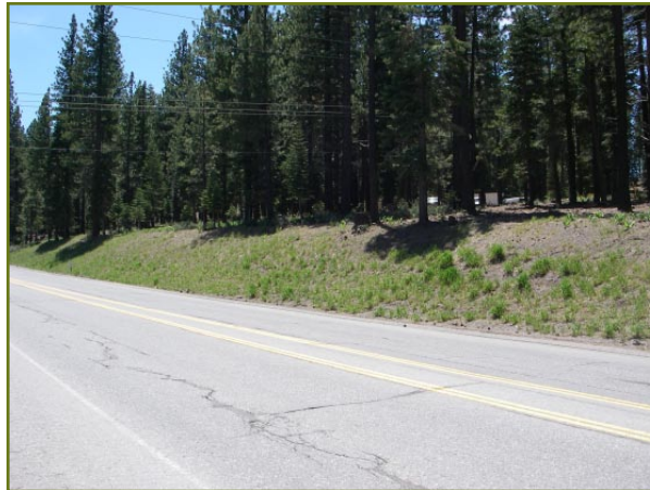
Highway 267 slope, three years after treatment.
