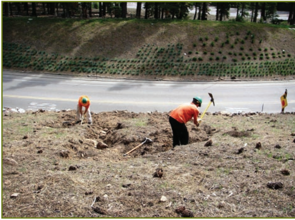
Loosening soil by hand using pick mattocks.
