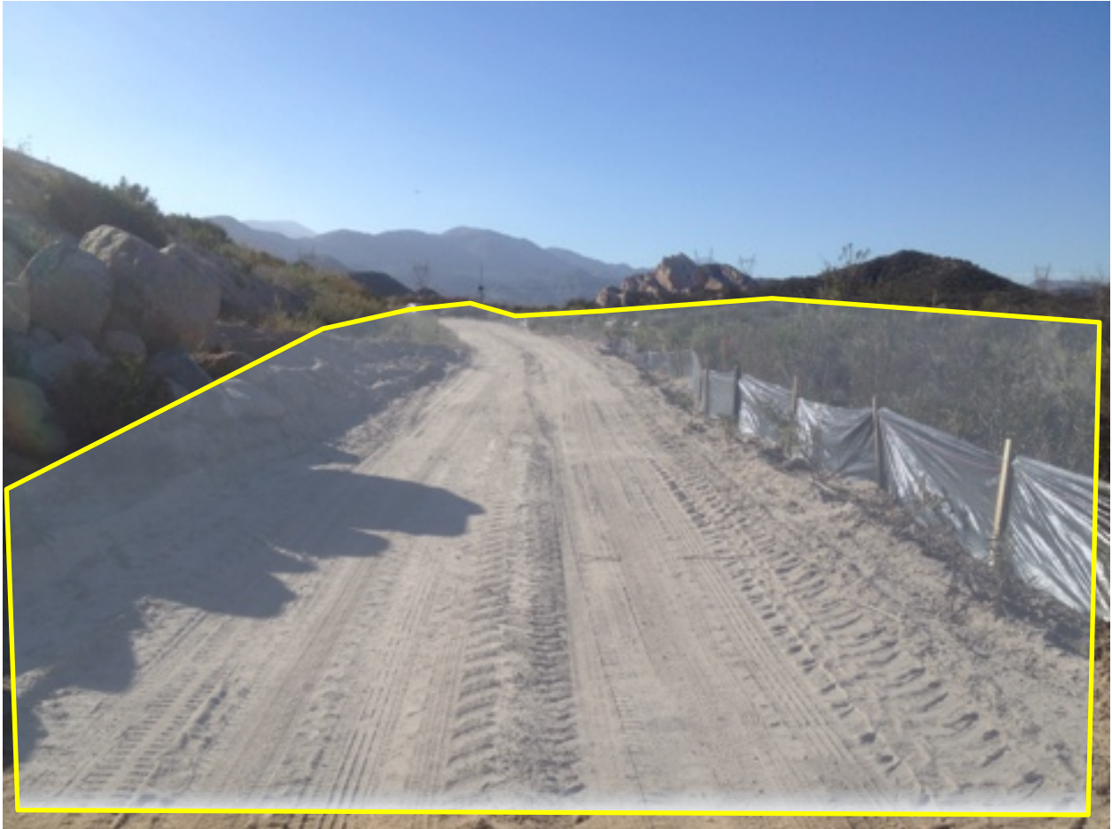
Picture 14: View West of silt fence installed as wildlife exclusion fencing in the Cajon Creek stream channel. Note the road in the channel and rock rip rap along the southern banks of the channel (rough outline of channel area in yellow).
