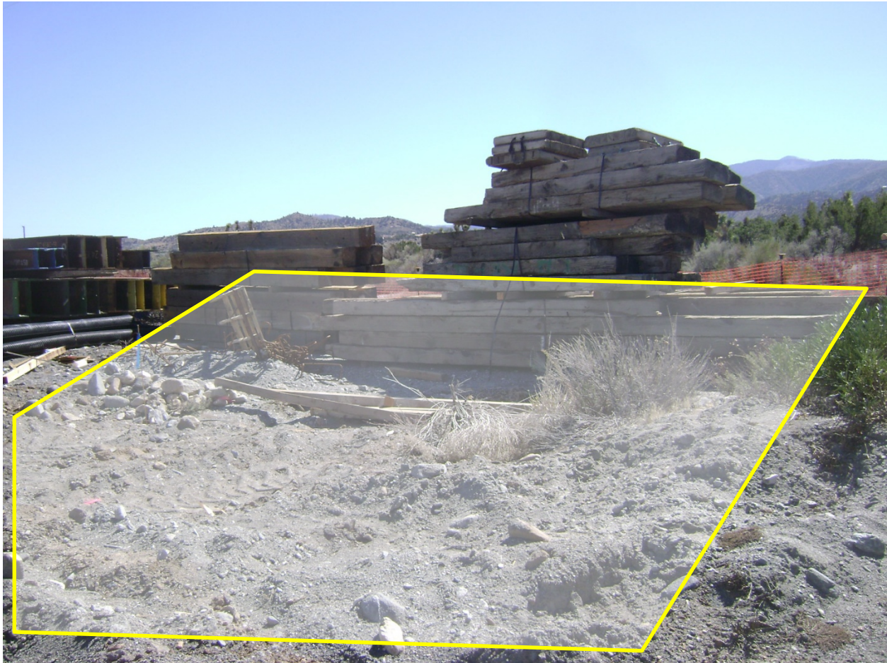
Picture 5: View South of timber mats stockpiled within the channel of Drainage I.D. 54 (rough outline of area in yellow).
