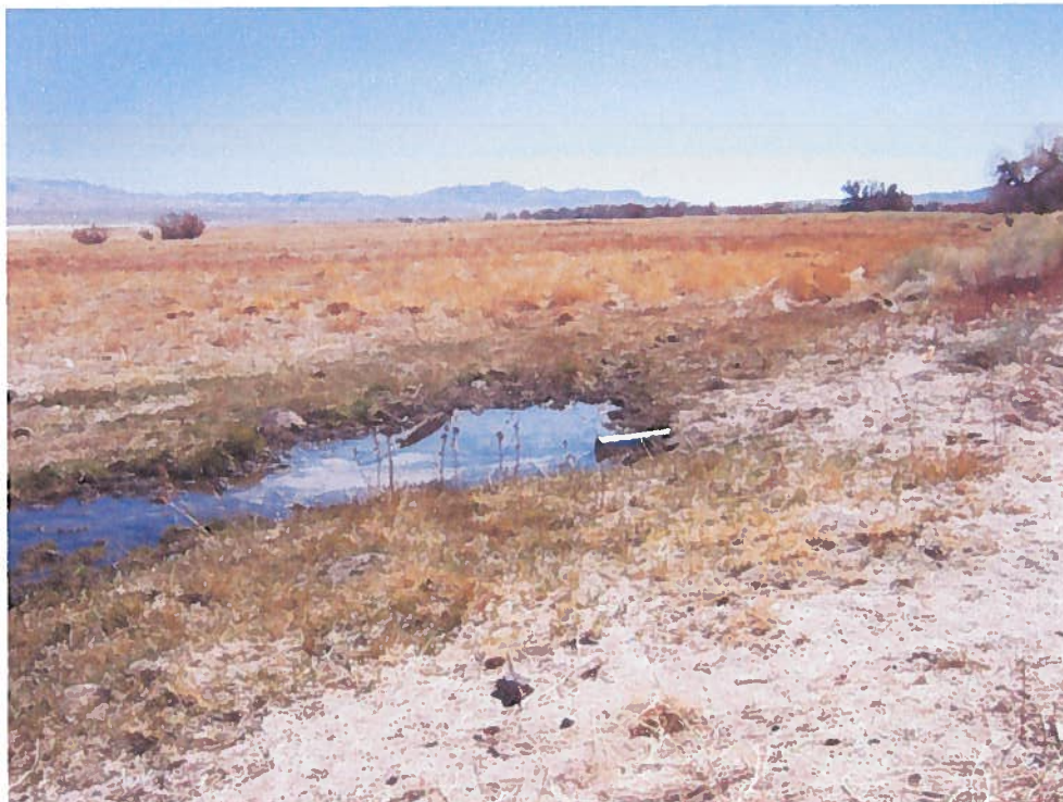
Photo 2 – View looking south at Fire Pond Outlet overflow discharge. Overflow from the Fire Pond is conveyed via an underground pipe and discharges to bare ground east of the facility in an adjacent wetland.
