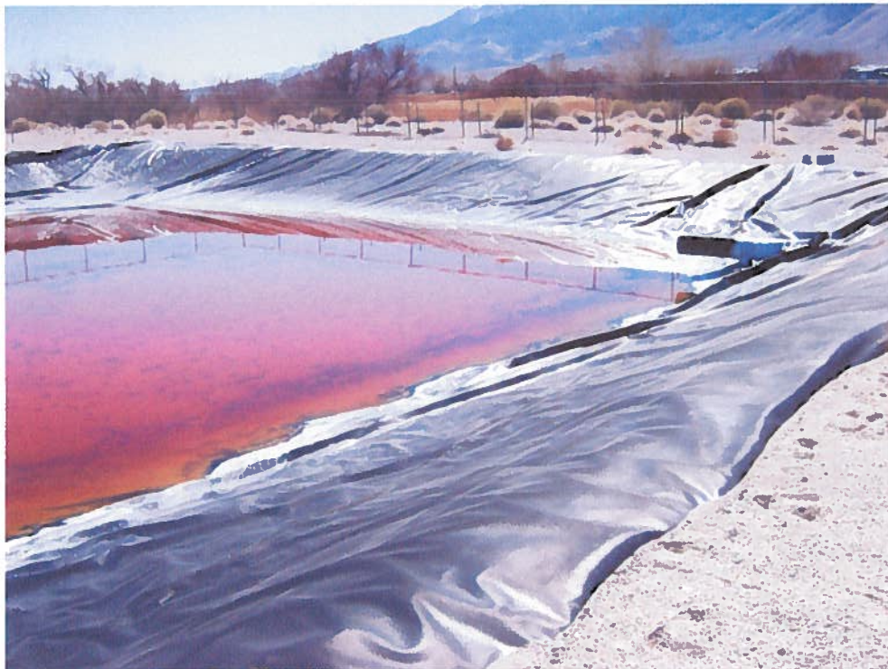
Photo 4 – View looking southwest across the Arsenic Pond . The pond receives wastewater from periodic regeneration and back-flush of the arsenic treatment system. Constituents of concern include arsenic and caustic soda.
