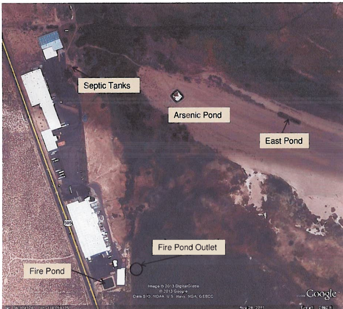
Figure 1 – Google Earth Aerial photograph of the Crystal Geyser Roxane facility and the waste discharge locations as described in the inspection report.
