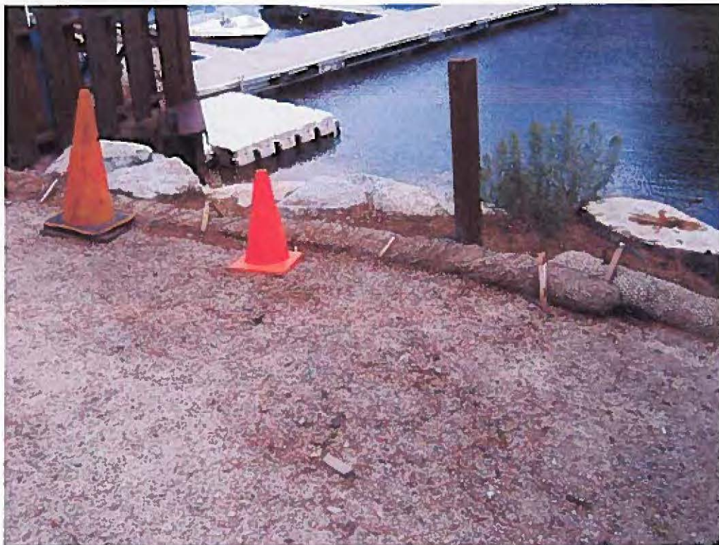
Photograph 06 - BMP joint is not J-hooked, and the fiber roll section by the pylons has been flattened. This area is by marina office, facing southeast
