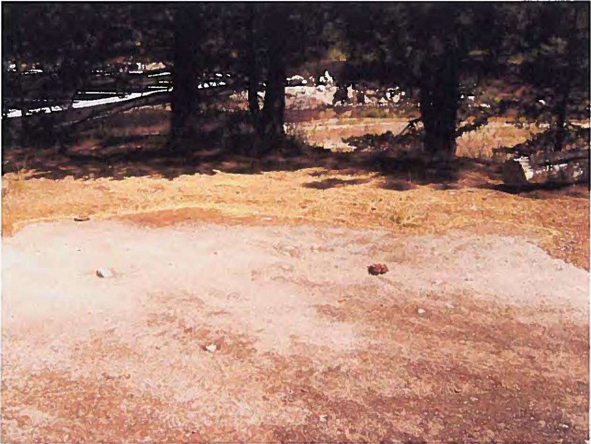
Photograph No. 33 – Close-up of storm water ponding line noted in Photograph No. 32. While there isn't evidence that stormwater runoff discharged over the bank in this area, it is likely that storm water flowed eastward toward the discharge point noted in Photographs No. 26-28.
