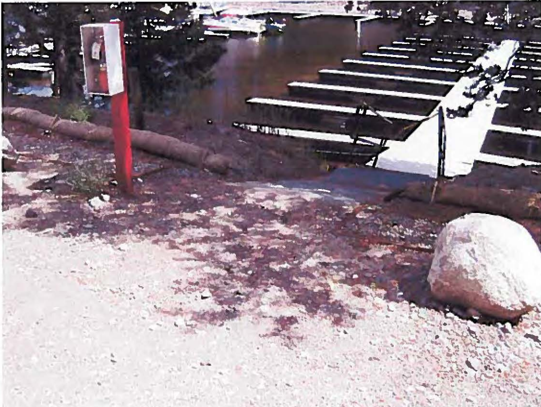
Photograph 09 – Close up of Photograph No. 08. Note that ends of fiber rolls are not J-Hooked.
