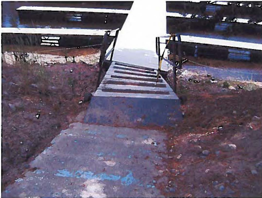
Photograph 11 – Moving closer to the second ramp west of office to get a further close up.
