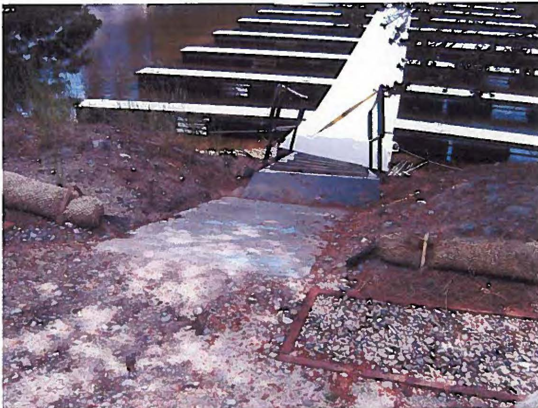
Photograph 10 – Moving closer to the ramp to get a further close-up of Photograph No. 08. Note that the fiber rolls do not prevent runoff from going down ramp and into marina
