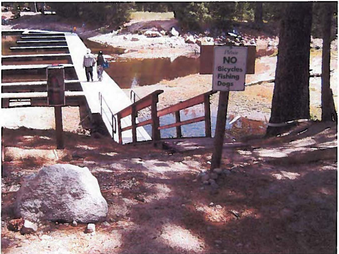
Photograph 20 - At 4th walkway ramp west of office. Fiber rolls to left of walkway and above walkway are not J-hooked at their ends. Fiber roll on right and above walkway is inundated with sediment, and evidence of sediment discharge into the marina is apparent.
