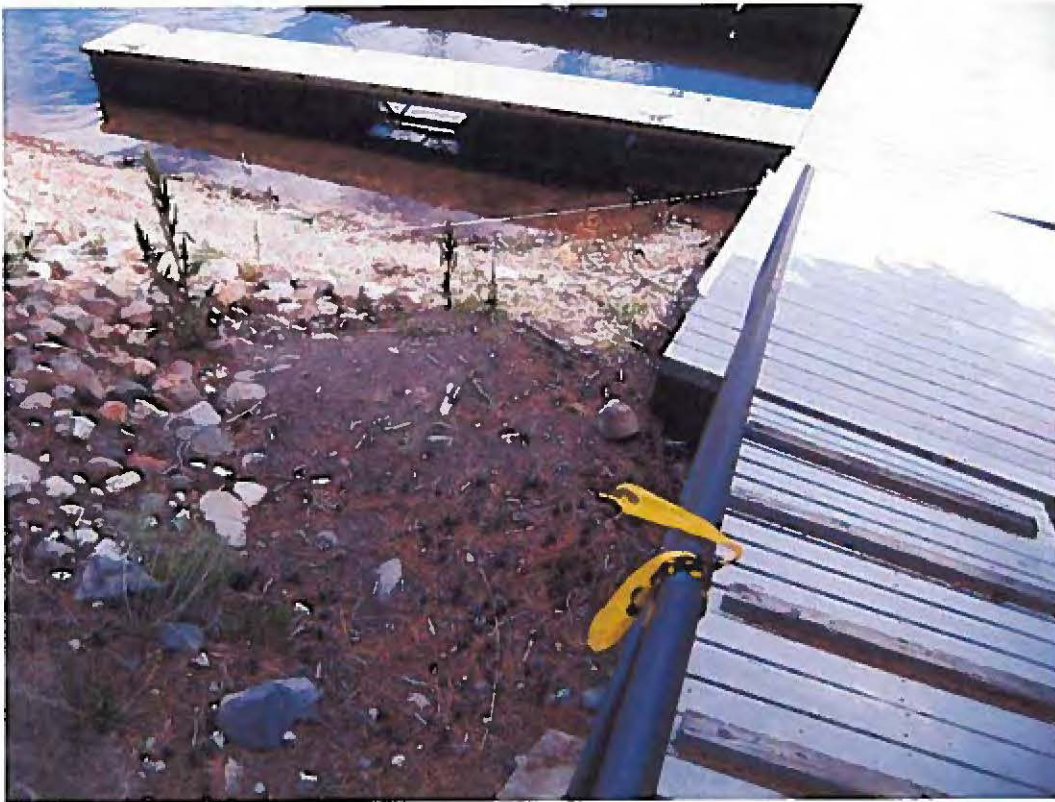
Photograph 13 – Close up of sediment deposit noted in Photograph No. 12.
