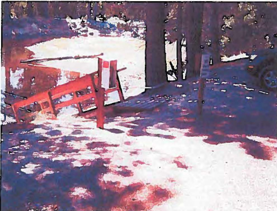
Picture 3: Gangway number three is also in a low depression of the hillside. These are potential sediment sources as there are no BMPs installed.
