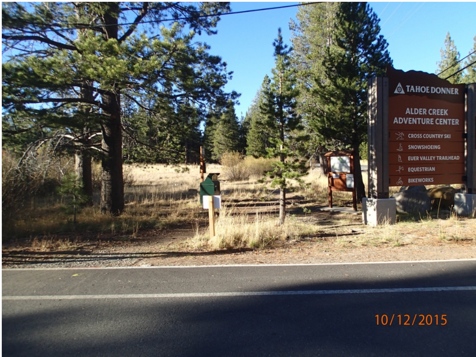
EXHIBIT 2: TDA EQ Sign Construction & Garbage Bin in Wetlands & 100 Yr Floodplain
