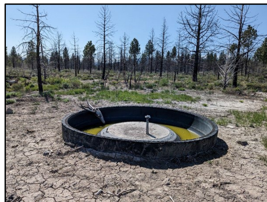
Recently installed upland water trough fed from a solar powered well on the Lassen National Forest's South Eagle Lake Allotment. This is a repurposed truck tire and is resistant to vandal bullets.
