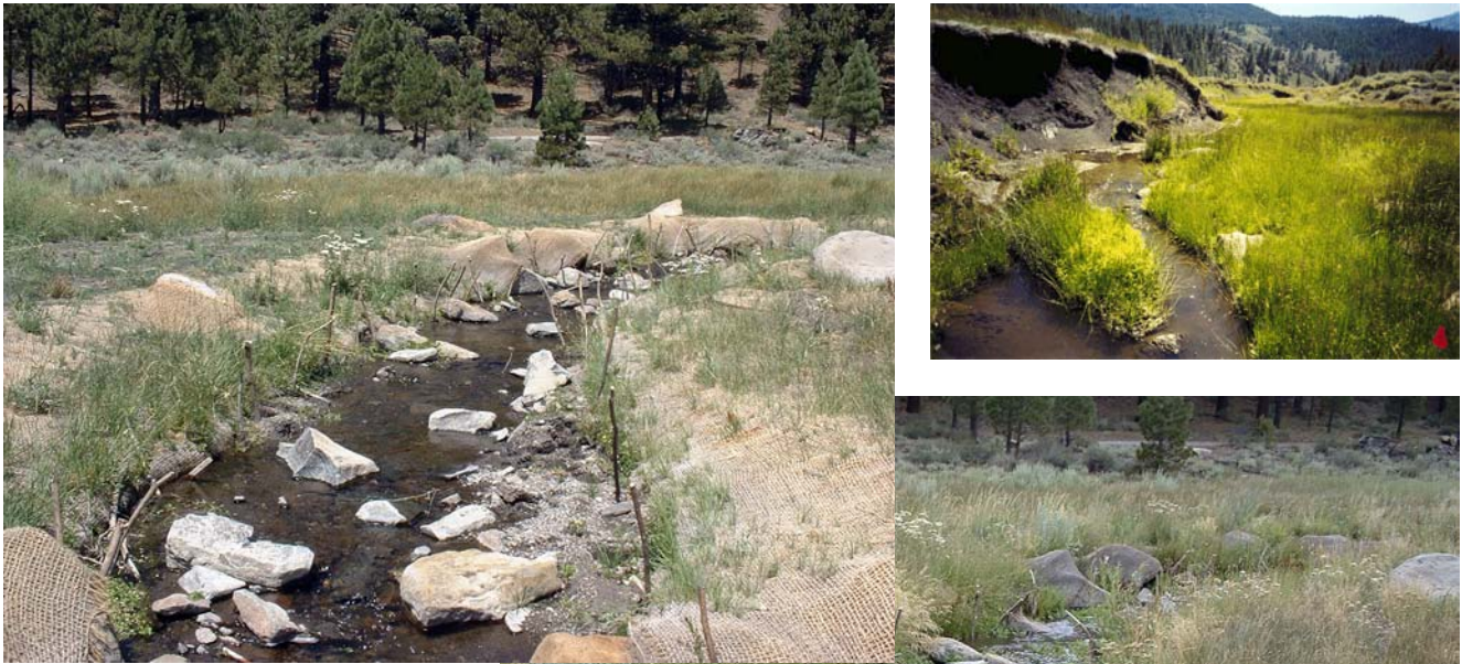
Fig. 2. Restoration of stream habitat in Bagley Valley Creek. The degraded, incised channel in 1999 (above right); the reconstructed channel upstream of the previous photo in 2002, the first year after restoration (above left); and the same location in 2003 showing extensive geomorphic and vegetative recovery (right). Photos by David Herbst
