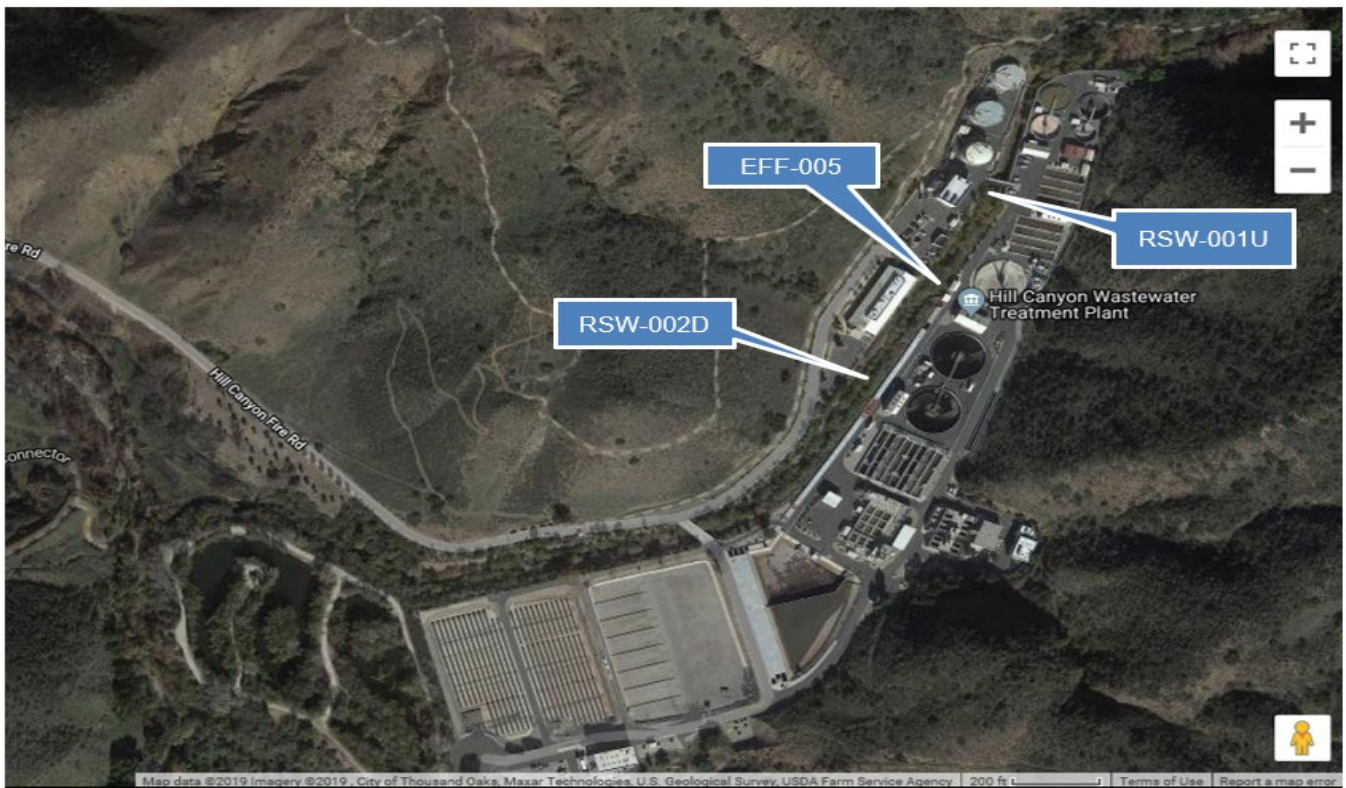
Figure E-1. Receiving Water Monitoring Station Locations RSW-001U & RSW-002D
