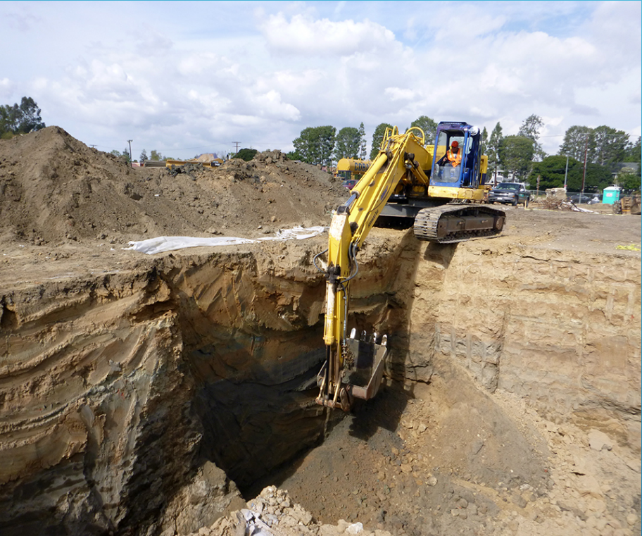
Soil Excavation Image from Gannet Fleming
