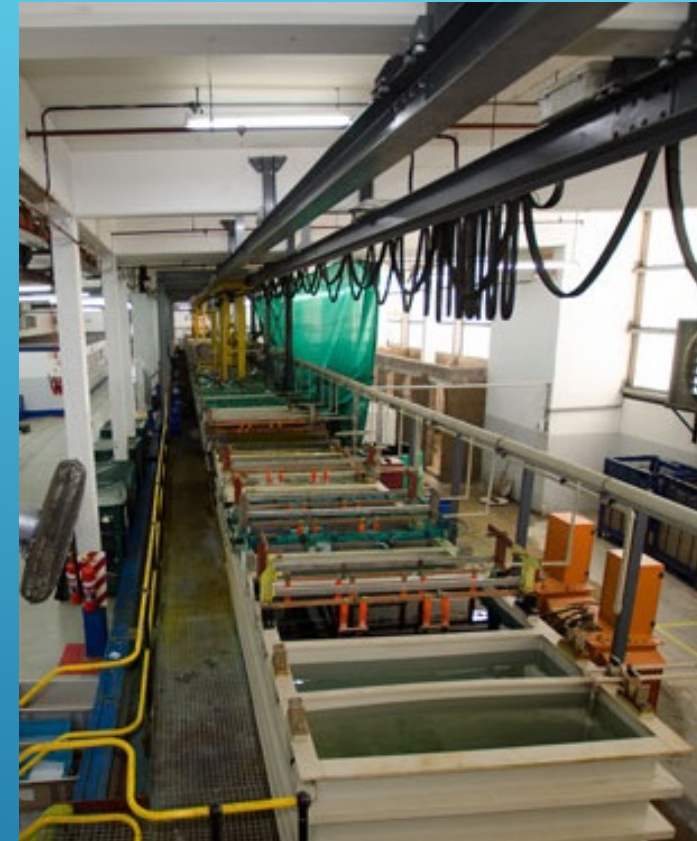
Commercial and industrial
