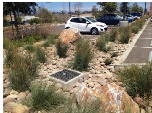
Figure 5-11 Recently Constructed Biofiltration in a Parking Lot
