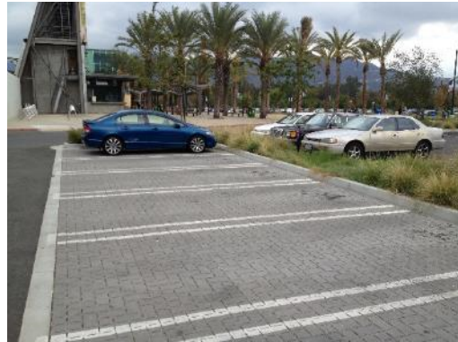
Figure 5-10 Bioretention and Permeable Pavement at the Los Angeles Zoological Park
