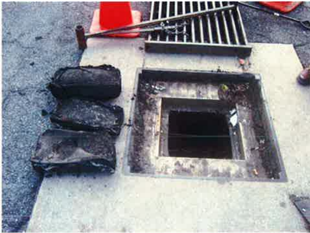
Figure 2. Used cellulose (front) and activated carbon (back) filters removed from HvdroKleen inserts after nine months service.
