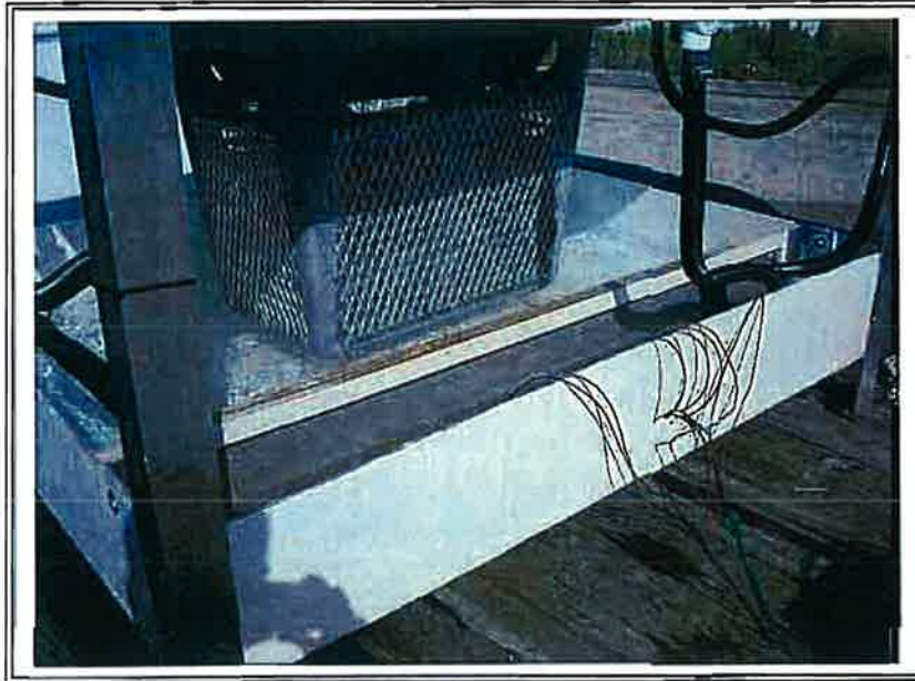
Photo No. 3: Grate Inlet Skimmer Box test bed, lower tier
