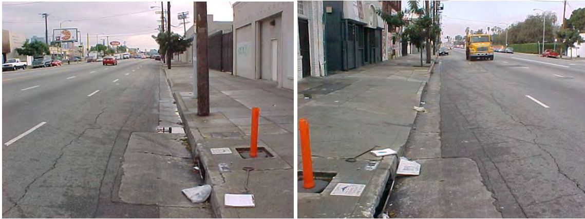
Figure 4-15. CC-001-H Site Photos Upstream (left) and Downstream (right).
