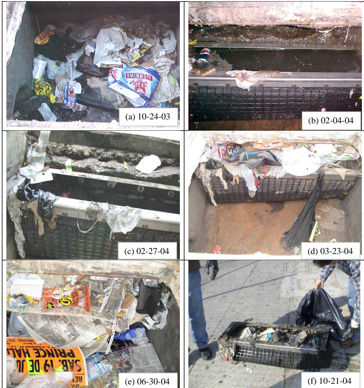
Figure 4-4. Field inspection photos of DrainPac catch basin insert at the intersection of Washington Blvd. and Vermont Ave.
