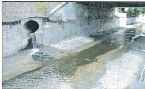
Outfall Discharging into Receiving Water
