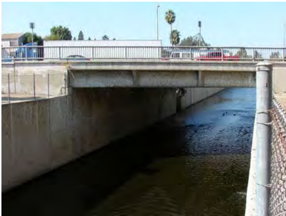
LAR_05_SEP Ground-Level View
