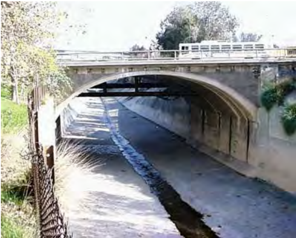
AS_SAN Ground-Level View
