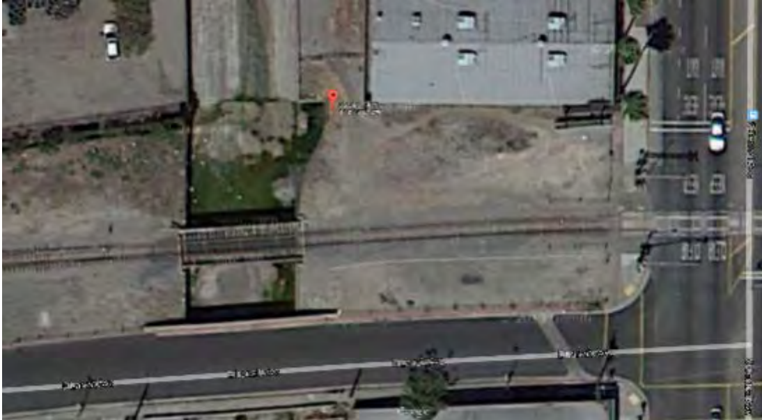
CC_SW_LAN Aerial View
