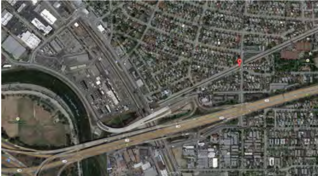
VW_CON Aerial View
