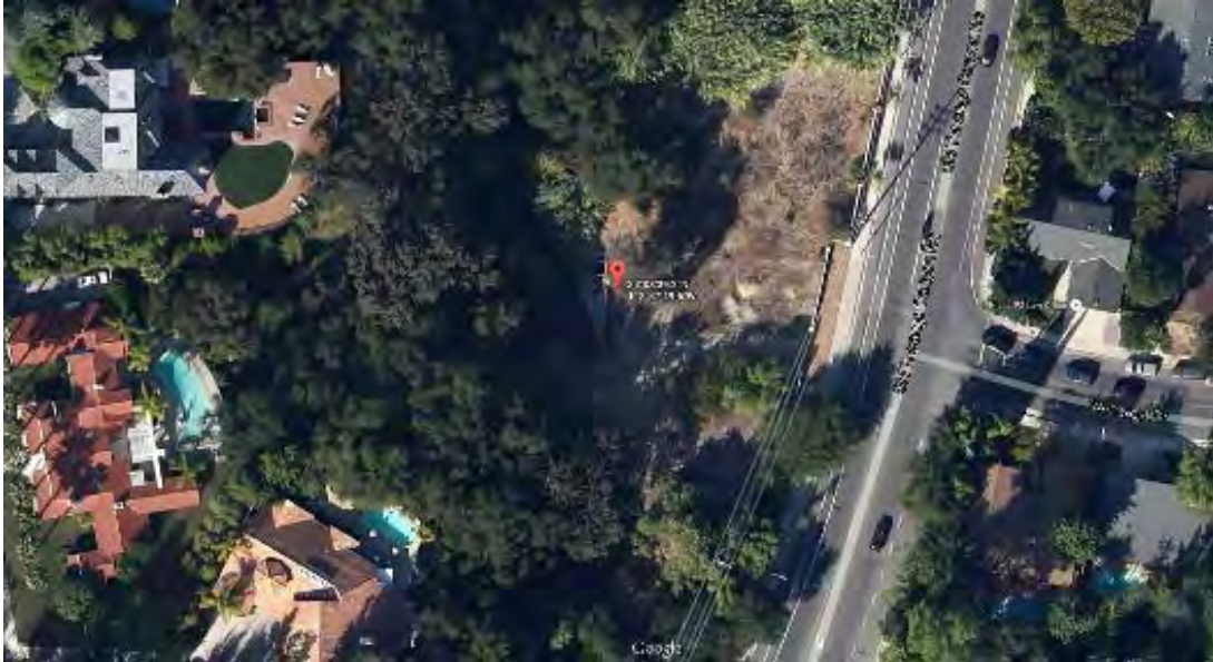
LAR_06_SW_OLD Aerial View
