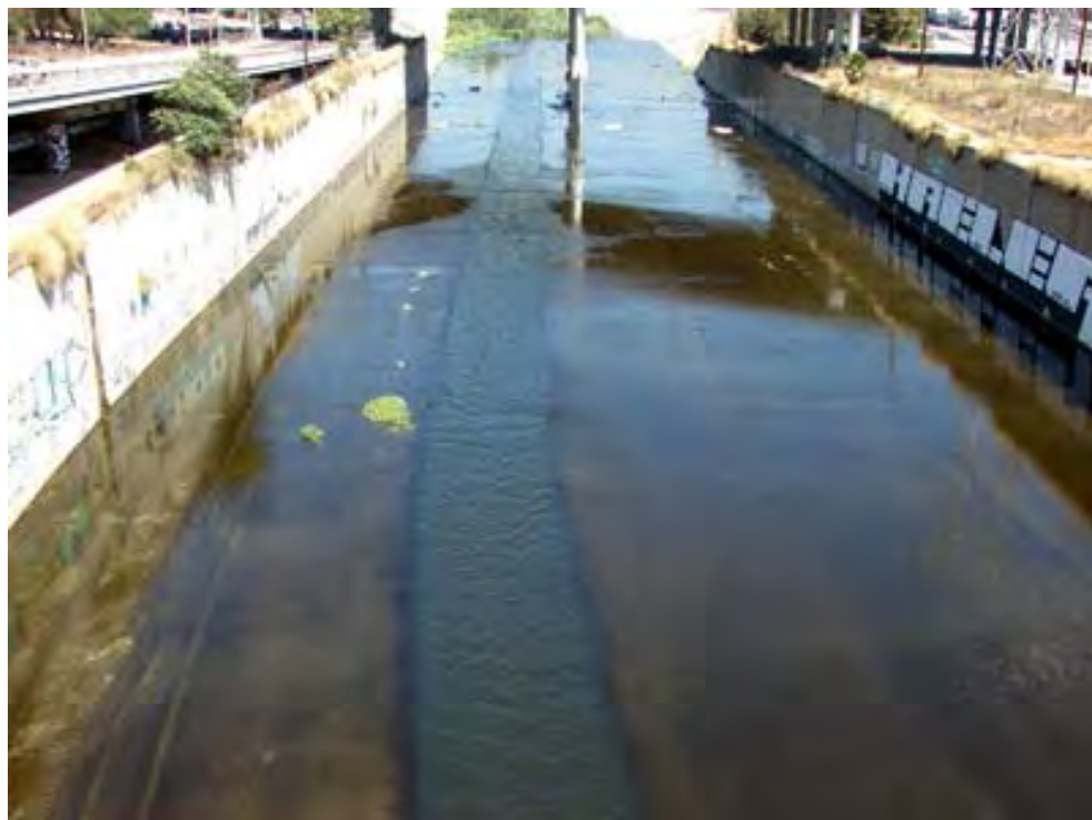
LAR_03_FIG Ground-Level View
