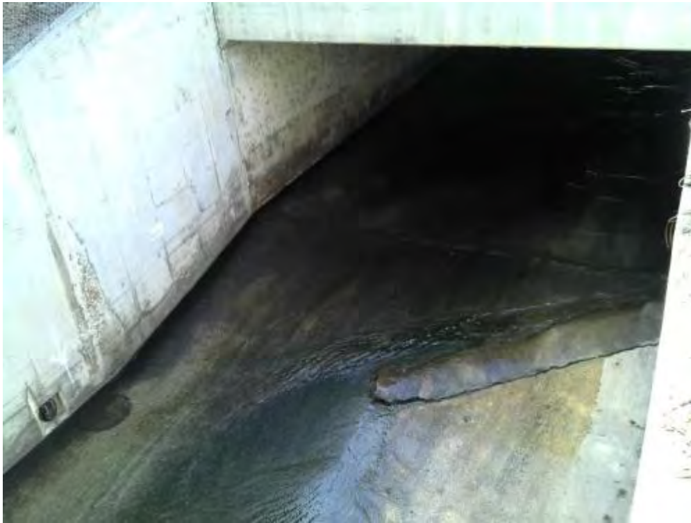
MCC_VAL Ground-Level View
