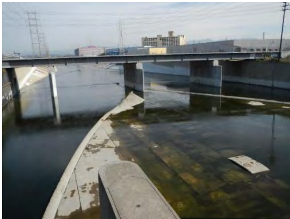
LAR_02_WAS Ground-Level View
