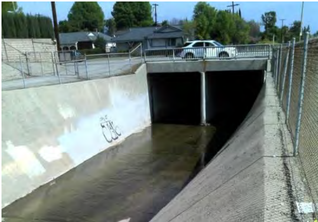
BEL_FAL Ground-Level View
