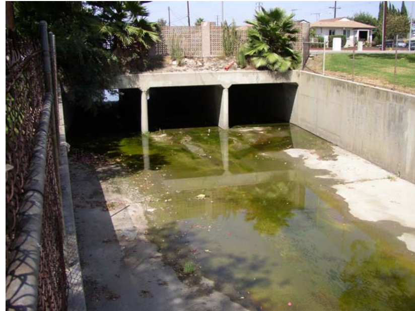
Figure 8. Dry Weather Flow in the Del Amo Channel showing Typical Dry Season Algal Growth found in Open Channels with Consistent Low Flows.
