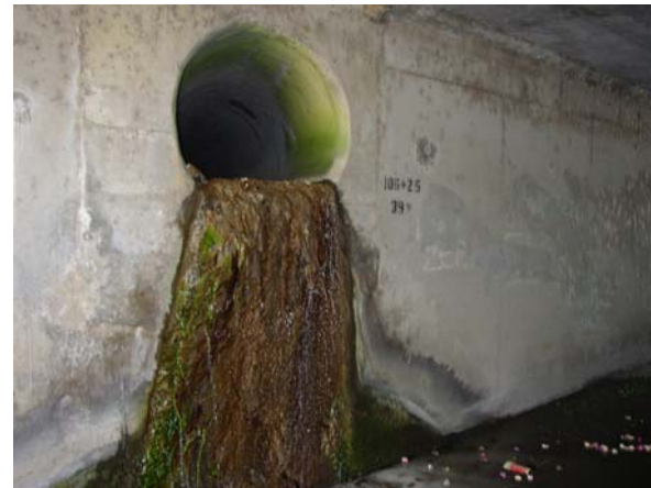
Figure 3. Concretions from Outfall into the Clark Channel under the Conant St. Bridge.
