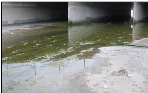
Figure D-1. Typical Dry Weather Flow Showing Algal Growth.
