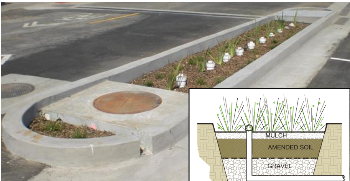
Figure 5-11: Example of Filtration BMP in Parking Lot 5 in Marina del Rey
