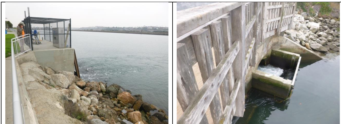
Figure 1-2. Tide Gate Separating the Grand Canal from MdR Harbor (Ebbing Tidal Conditions)
