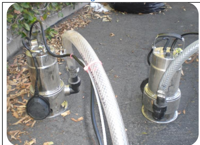
Submersible Pumps used to sample storm water from a well into the filtration units
