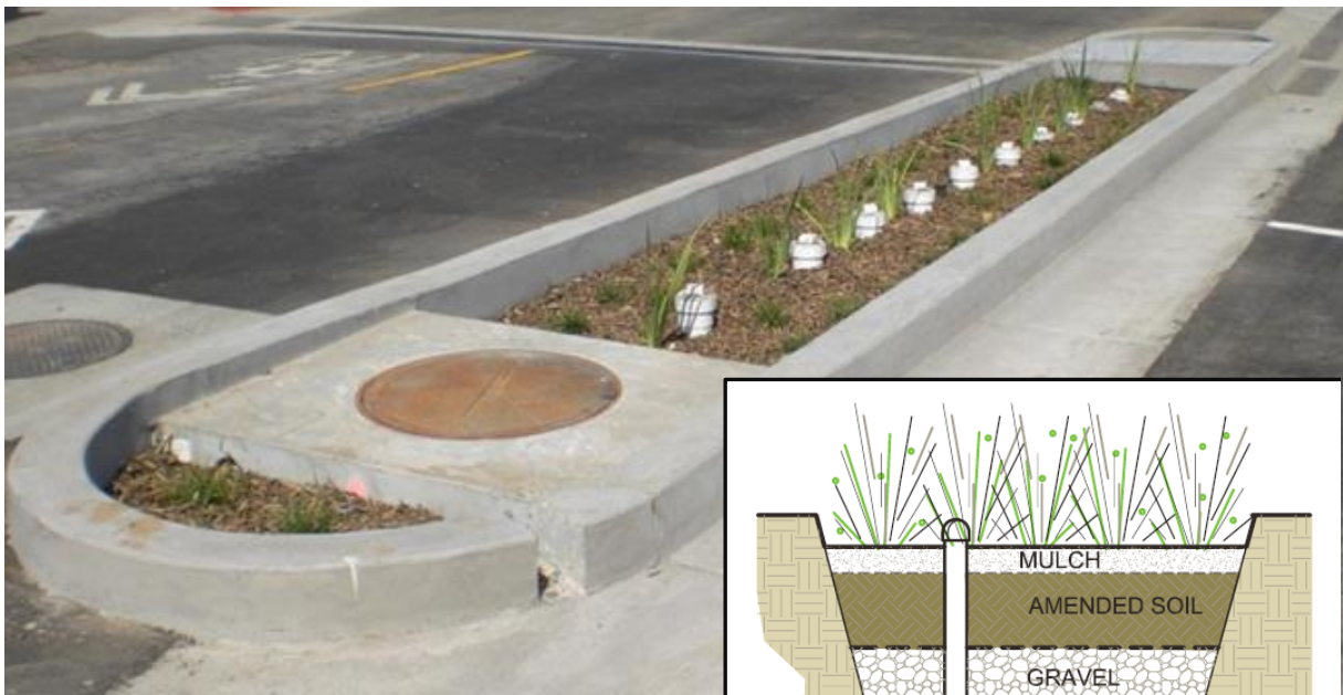
Figure 5-10: Example of Filtration BMP in Parking Lot 5 in Marina del Rey
