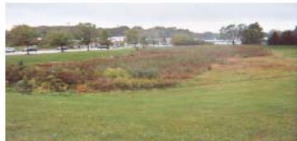
Figure 1. Example of a Dry Extended Detention Basin
