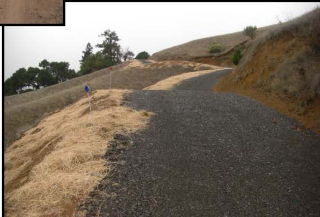
RE-GRADED OUTSLOPED ROAD WITH ROLLING DIPS
