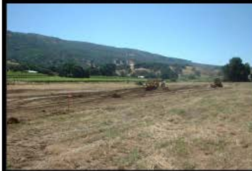
Grading for 2002 project
