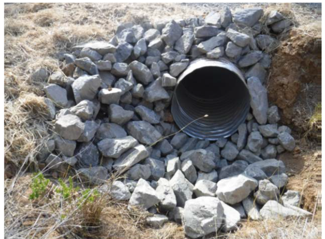
Image 3: Outlet of replaced culvert with scour repaired and erosion potential diminished.
