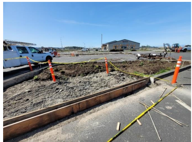
LID Basin B during construction (photo taken on March 12, 2023).
