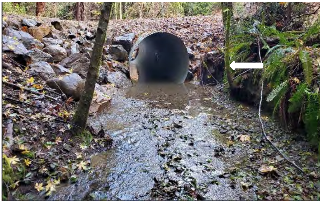
Figure 6. After culvert replacement—a larger culvert has been placed at the proper elevation to allow stream flows and materials to pass through unimpeded.
