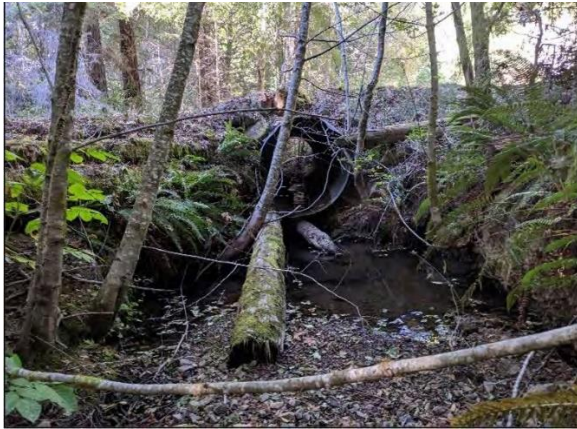
Figure 6. After culvert replacement—a larger culvert has been placed at the proper elevation to allow stream flows and materials to pass through unimpeded.
