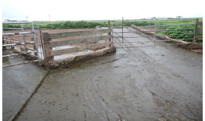
Concrete lanes and concrete curbs help control manure runoff and assist in the daily maintenance of the ramp to the manure pond. Humboldt County. Photo by Cherie Blatt
