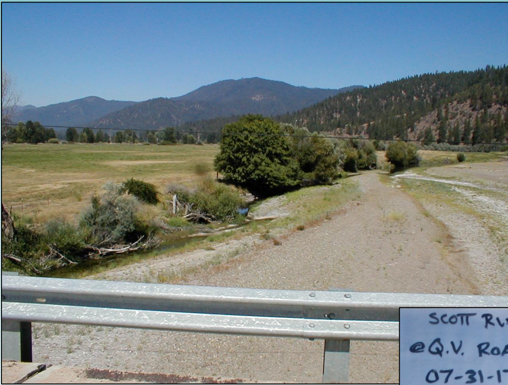
Quartz Valley Road Bridge August 13, 2001
