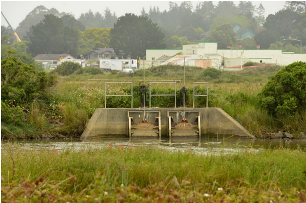
Figure 11: One of the Main Restoration Components in Area 1 is the Removal of Existing Tides Gates to Allow Tidal Inundation of the New Channel System. Removal of Barriers Such as this Will Increase Habitat for Fish and Aquatic Species
