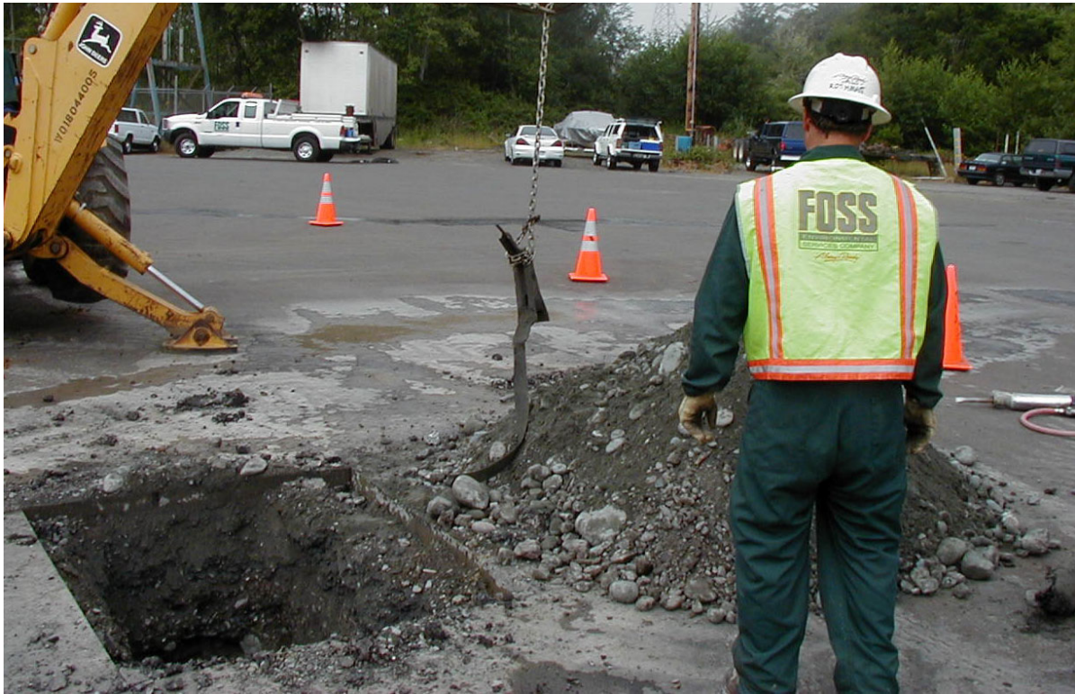
Photograph 9 – Shows the limited excavation at Anomaly C.
