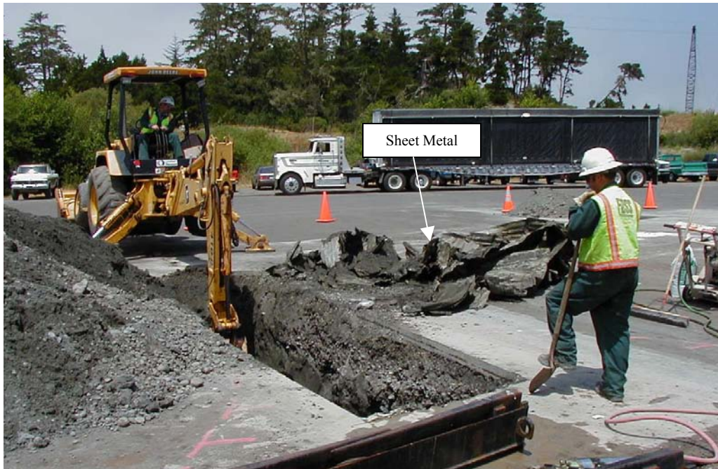
Photograph 6 – Shows sheet metal removed from the excavation at Anomaly A.
