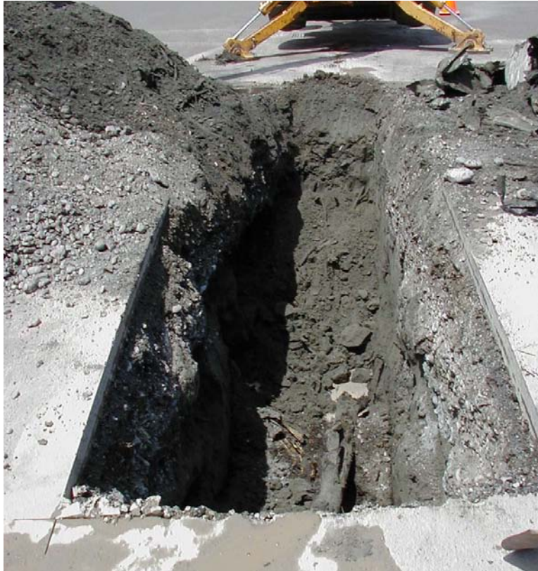
Photograph 5 – Shows the limited excavation at Anomaly A.
