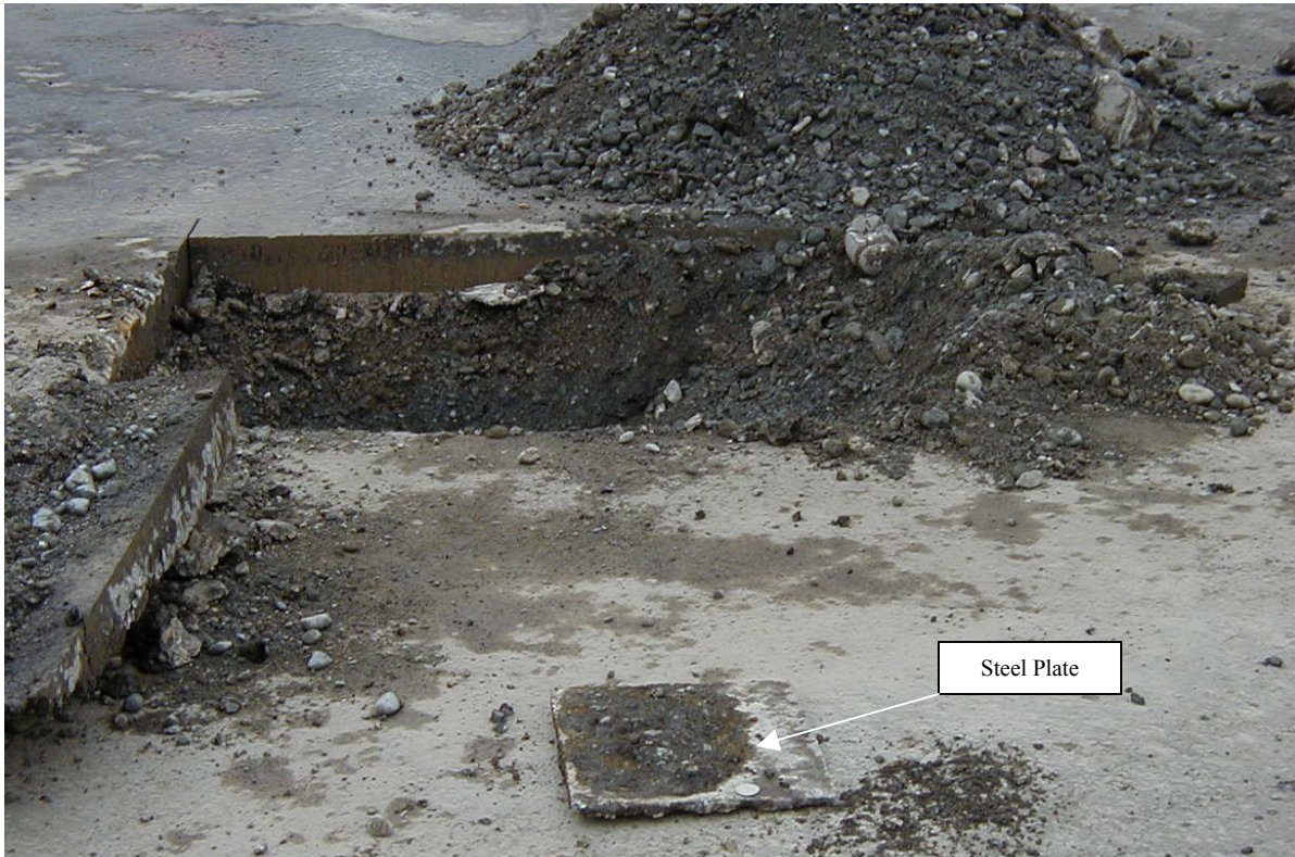
Photograph 11 – Shows the limited excavation at Anomaly D and the steel plate removed from the excavation.
