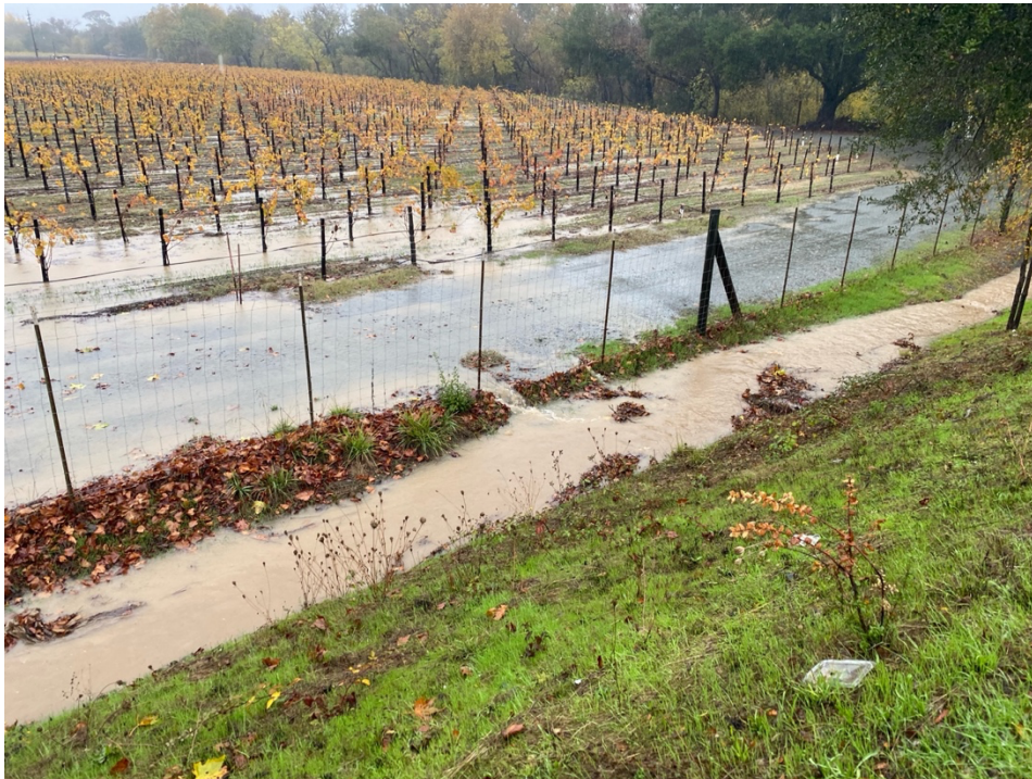
Image 1: This picture was taken in the most recent storm event November 21, 2024 and is of a vineyard with less than 10% slope. Per the Proposed Order, this vineyard would need a minimum of 50% groundcover by December 15 to address sediment discharges and linear sediment controls prior to a Qualifying Storm Event when ground cover minimums are not yet met. Looking at this particular instance, the 50% groundcover minimum appears to be about met and thus, no linear sediment controls required even though they would be more protective of water quality.
