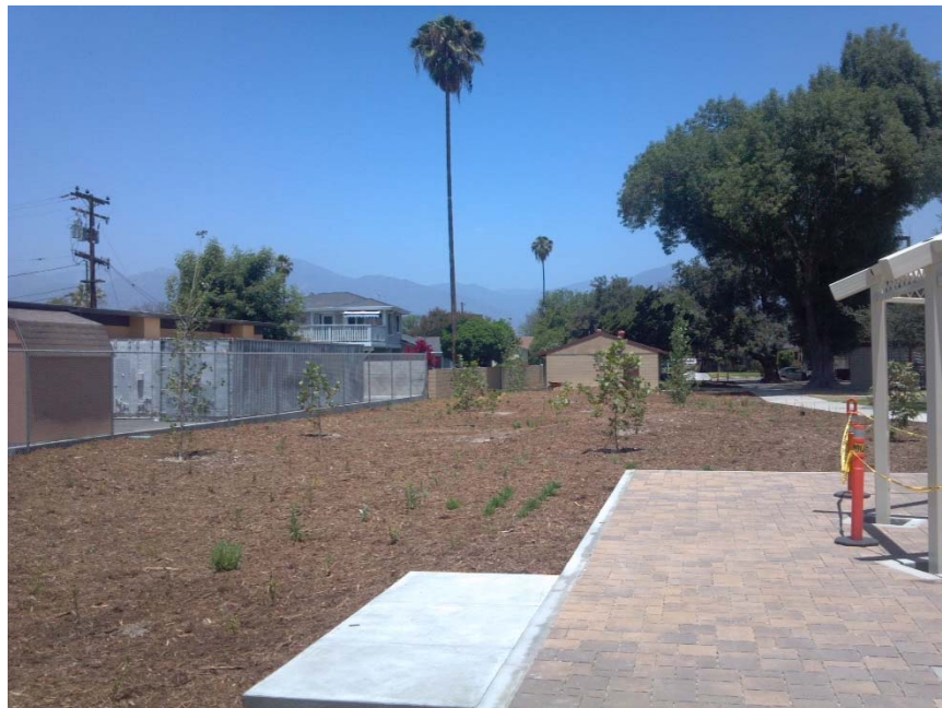
Mulched infiltration swale at Lambert Park
